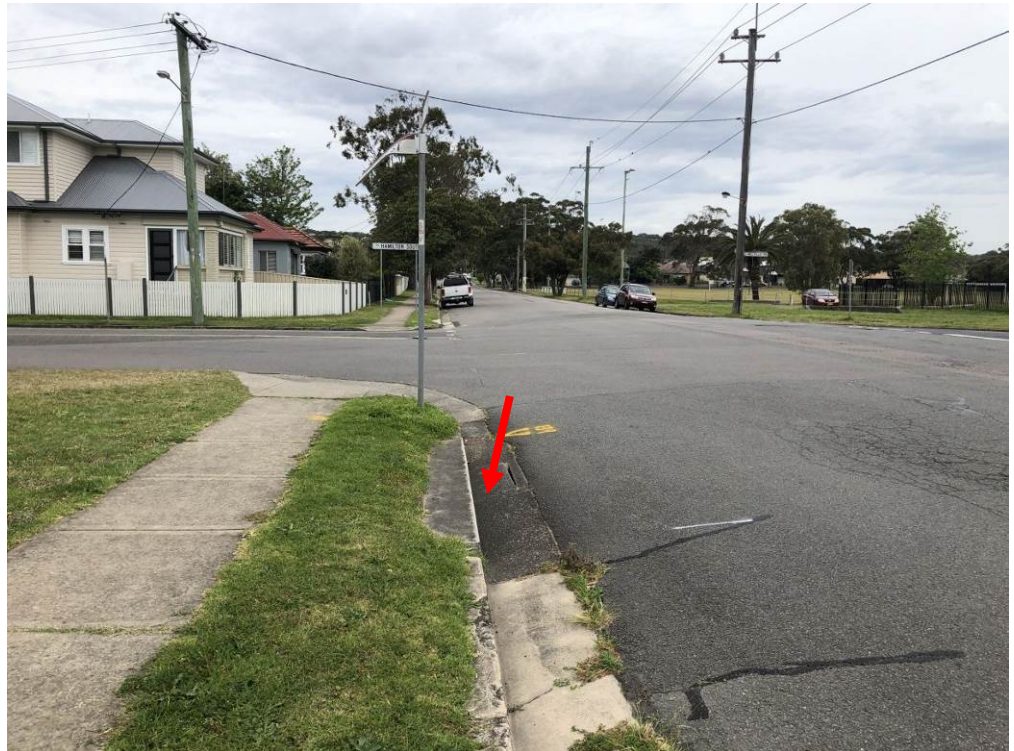
Photograph 3: Existing Pit “ExP4” in Chatham Street
