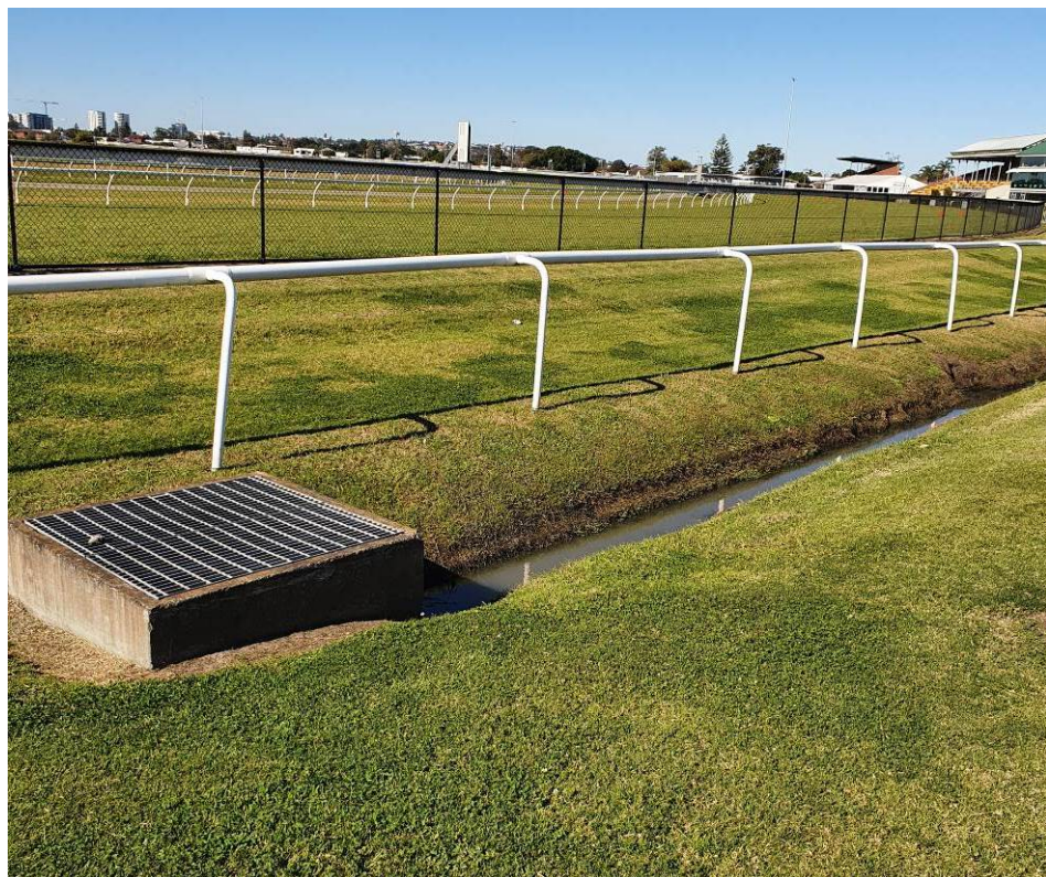
Photograph 6: Existing Pit “ExP7” Adjacent to the Track
