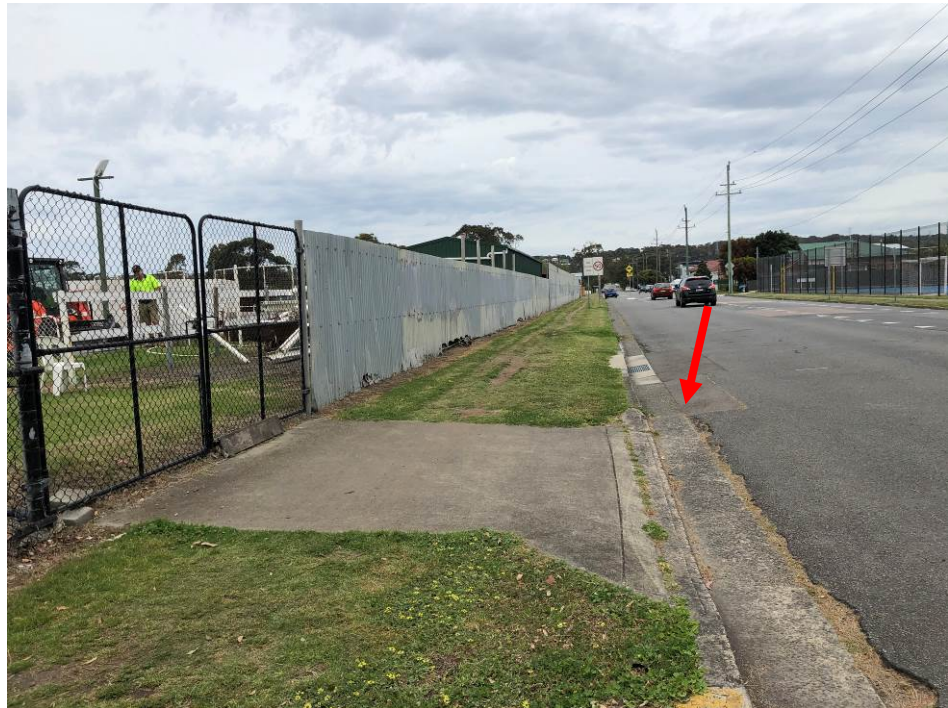
Photograph 5: Existing Pit “ExP6” in Chatham Street
