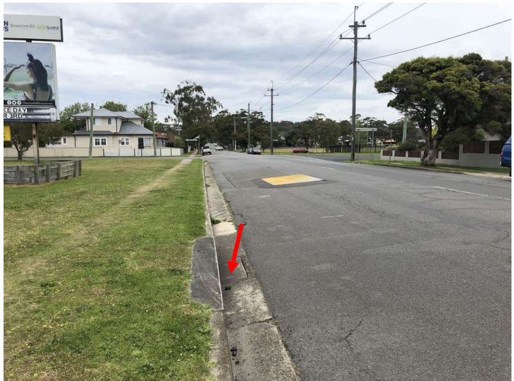
Photograph 4: Existing Pit “ExP5” in Chatham Street
