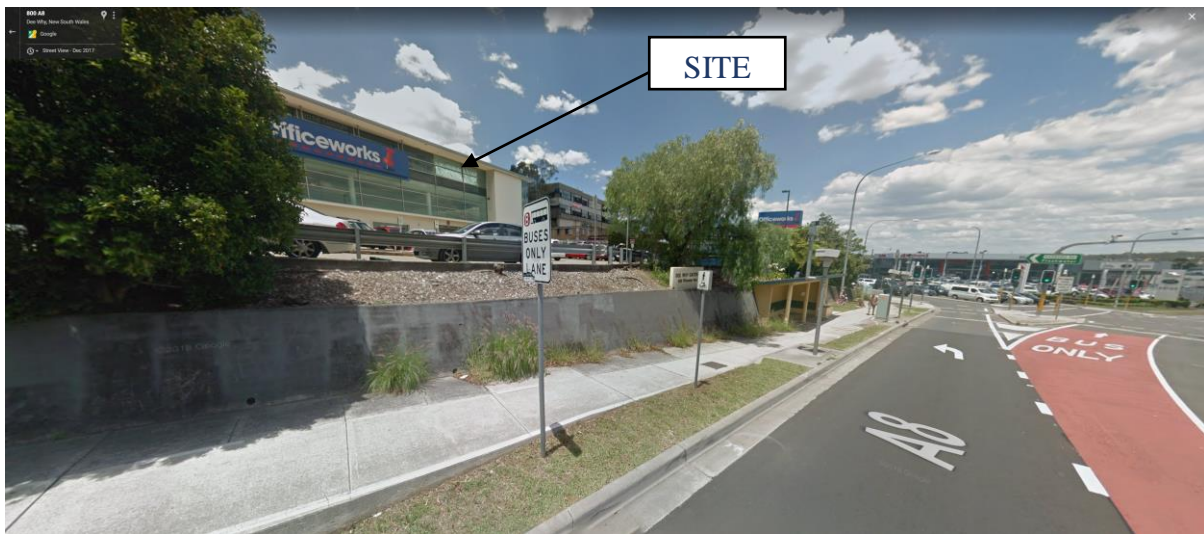
Figure 12: Shared Path on Pittwater Road looking southbound
