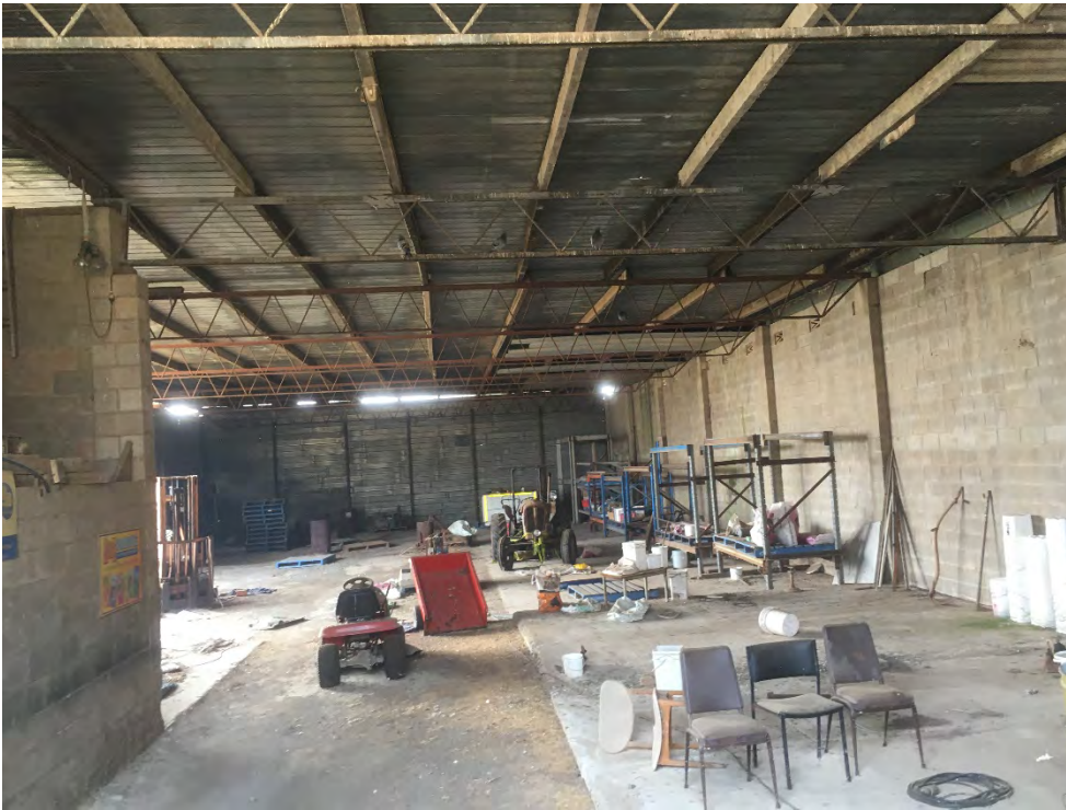
Photograph 5.7 Inside of disused farm shed showing metal truss and roofing
