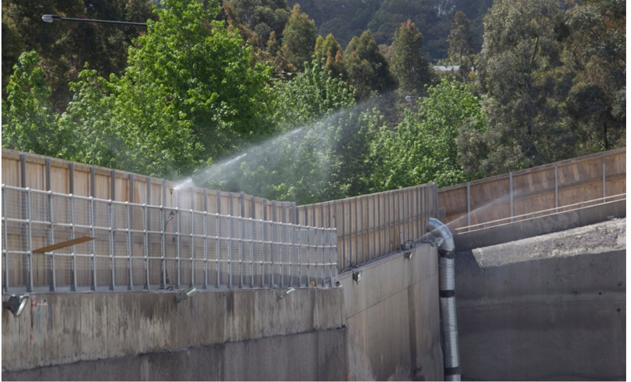
Figure 8 Dust Mitigation at Northwest Station Site
