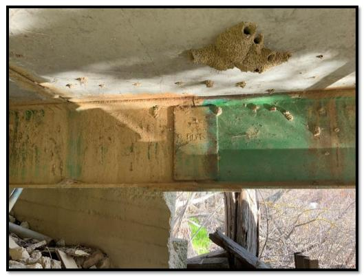
South abutment: accumulated dirt and rust on I-Beam
