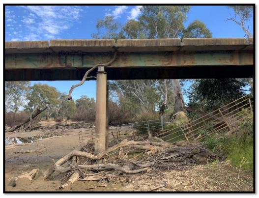
Nth bank looking from east side of bridge: old farm gates, accumulated debris and a branch jammed in the superstructure – refer above and below
