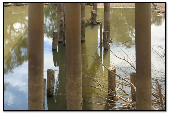
Waterway: old timber piles act as obstacles to flow, adding to accumulation of debris
