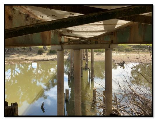
Diagonal bracing between I-Beams provide lateral support
