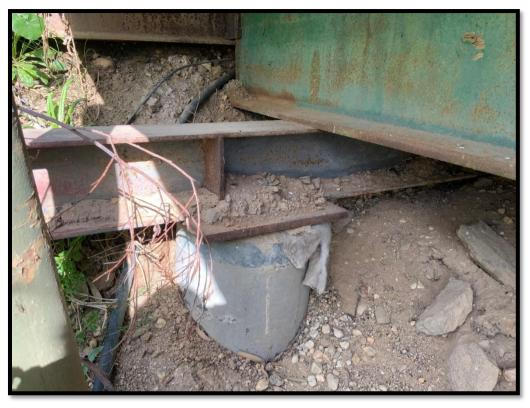
South abutment: crosshead resting on steel plate / packer - refer above and below
