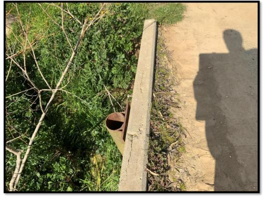
SE corner of bridge: cracked kerb. Old guide post was previously cut / removed
