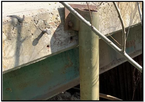
SE corner of bridge: crack in previous image extends down side of kerb. This damage was possibly caused by vehicle impact
