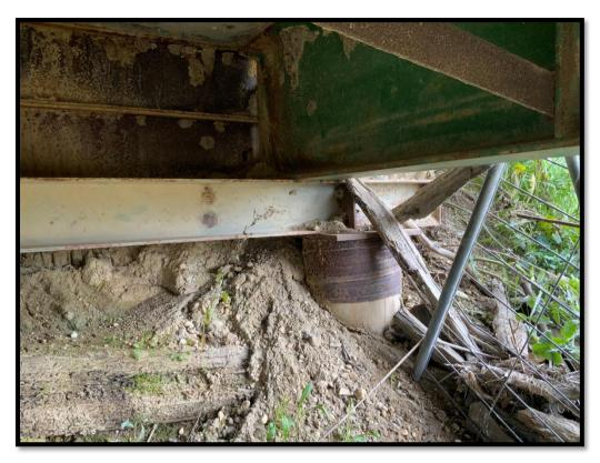
North abutment: quasi fender wall assists in retaining soil on the embankment – refer above and below
