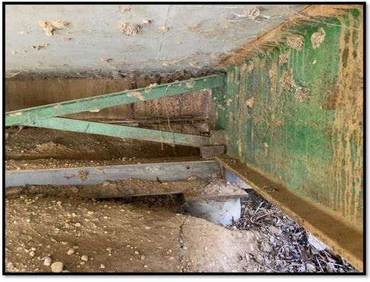
Steel throughout Bridge structure is coated with rust and dirt / silt – refer above and below
