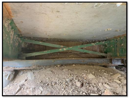
South abutment: steel fender wall behind the crosshead and diagonal bracing
