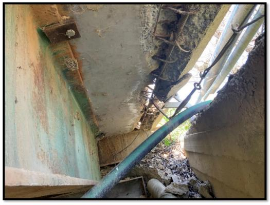
SW corner: broken kerb and exposed reinforcement viewed from beneath
