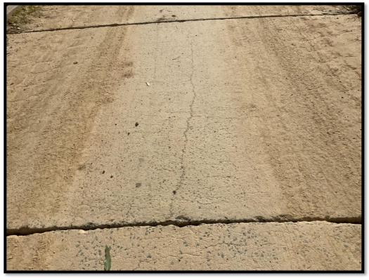
Deck: cracks visible in deck units are not active
