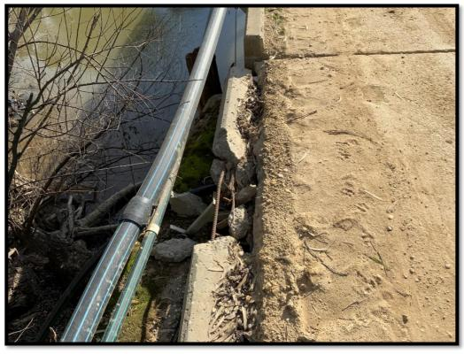
SW corner: broken / separated kerb and exposed reinforcement – refer above and below
