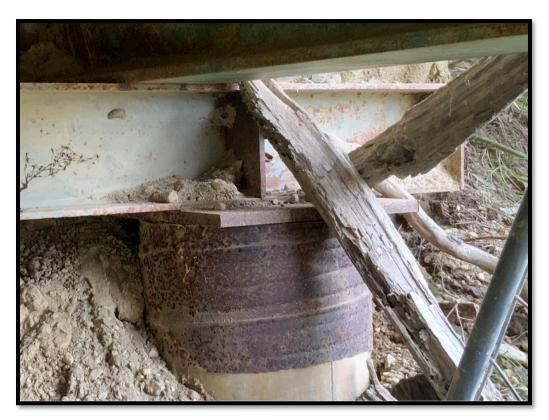
North abutment: both piles have been extended (note different colour), levelling plate / packer at top of pile, web stiffener near each end of crosshead
