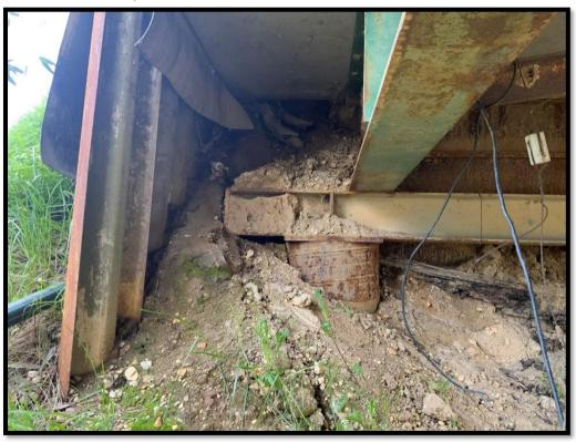
North abutment: note 'w-beam' embankment stabilisation on LHS of image
