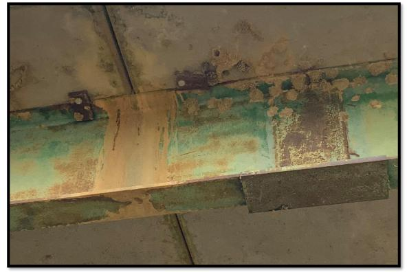
I-Beam: fastening securing the deck unit to the I-Beam is loose, and has moved out of position. Also note the prevalence of rust / dirt
