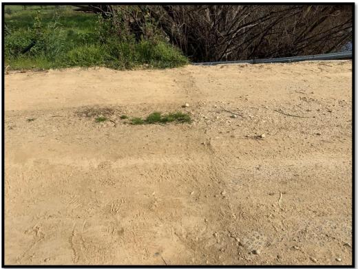
Approach: depression / slope has formed in front of the first deck unit
