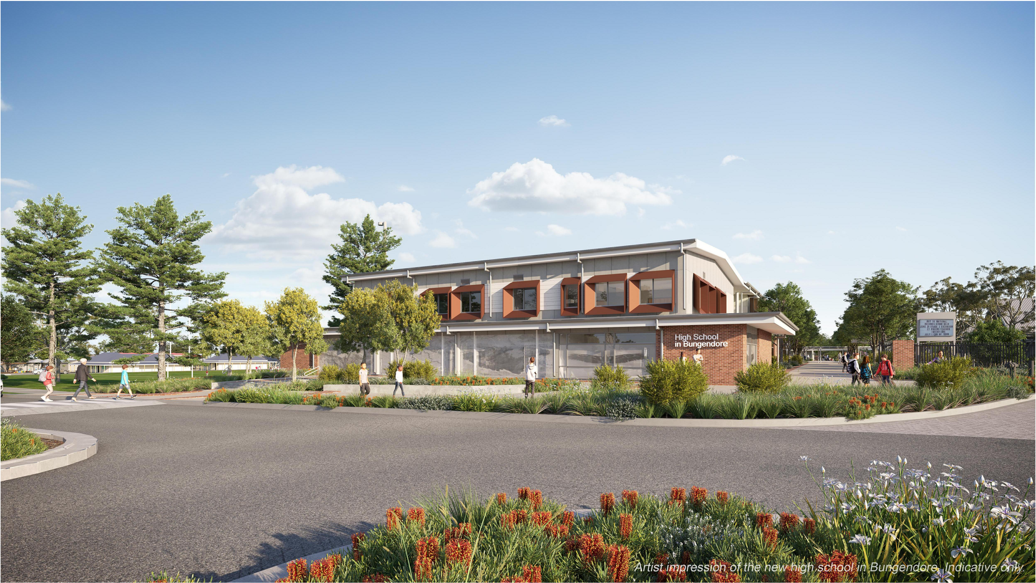
ENTRY FORECOURT FROM MAJARA STREET
