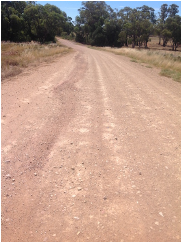
Wilmartha Road surface between Fifield and Sunrise Lane
