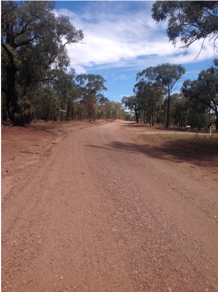
Wilmartha Road junction of Sunrise Lane facing South towards Fifield.
