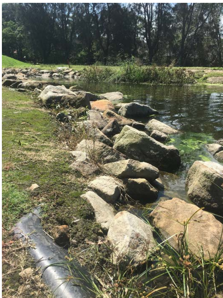
Figure B5-3 Cammeray Golf Course dam edge with exposed plastic lining, sandstone rock and fringing aquatic vegetation
