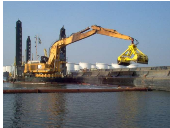
Figure 5 Example environmental clamshell in operation (source: Boskalis)
