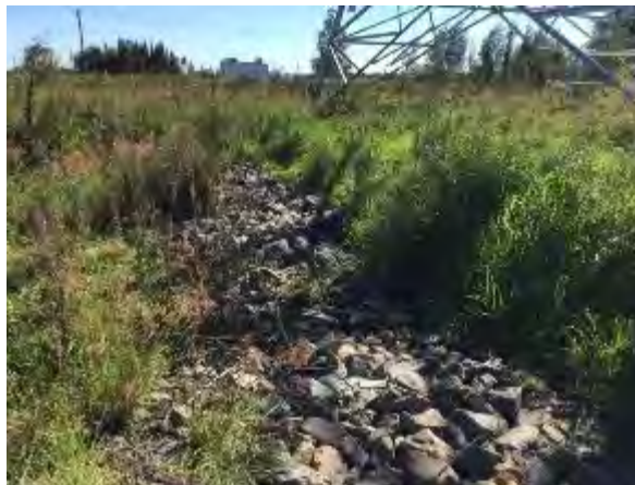
Photograph 7.14 Drainage line, SU3, view to west (ERM 2019)
