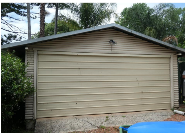
Figure 3.20 The c.1960s garage to the eastern boundary which has likely been upgraded at some stage.
