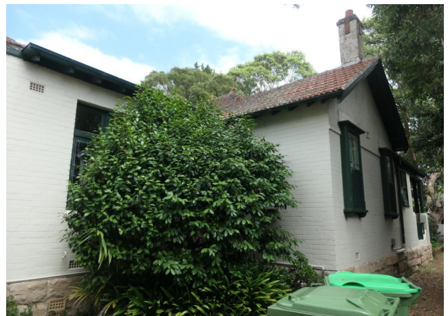
Figure 3.19 Eastern elevation of 37 Bancroft Avenue where the sandstone footings are visible and some original windows remain to the front portion of the house. The windows to the rear are later.
