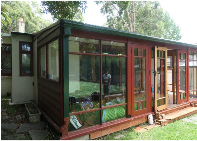
Figure 3.22 The late twentieth century rear sunroom enclosed with windows and doors.
