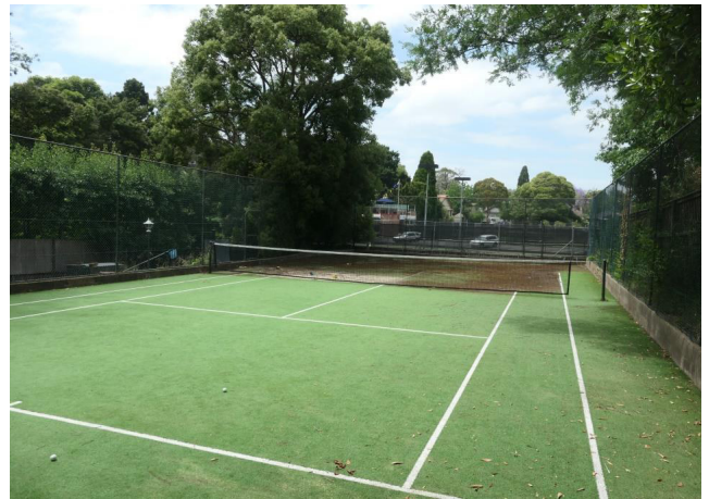
Figure 3.25 The late 1930s tennis court in the rear yard, resurfaced in 1988.
