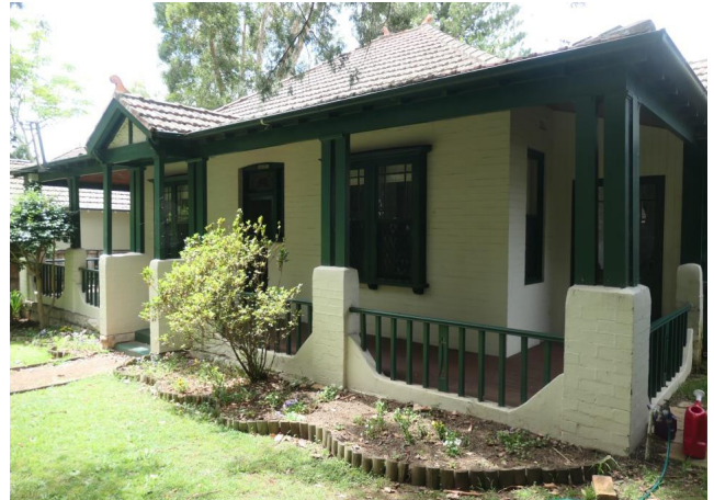
Figure 3.17 Front facade of 37 Bancroft Avenue. The facebrick has been painted white and the verandah balustrade has similar infill treatment as the front fence.
