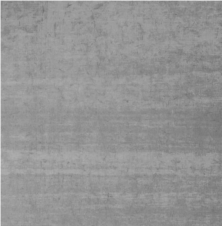
OFF-FORM CONCRETE (CO1)
