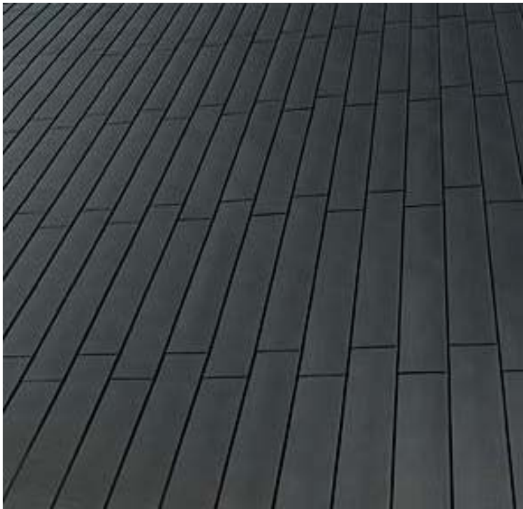
VERTICAL JOINT CFC CLADDING PANELS (CFC2)
