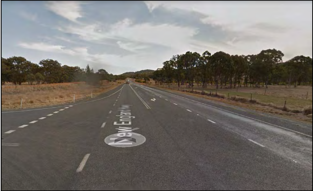
Photo 2 – Sheltered turn lane for right turning vehicles into Sunnyside Platform Road from the New England Highway. Note straight alignment that allow for good visibility
