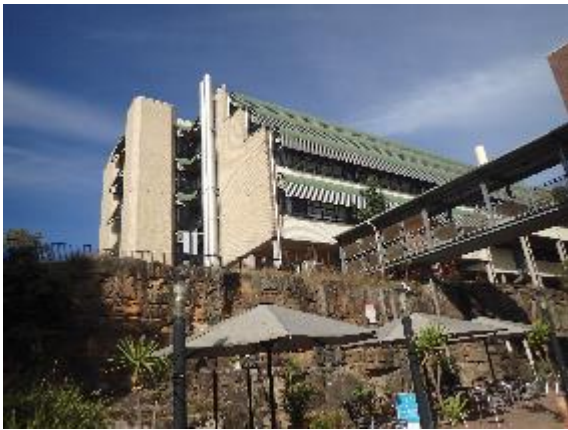
Figure 5.1 Northern aspect of building J. Note the curved window awnings and the staggard brick siding. Also note the sandstone cliff face.
