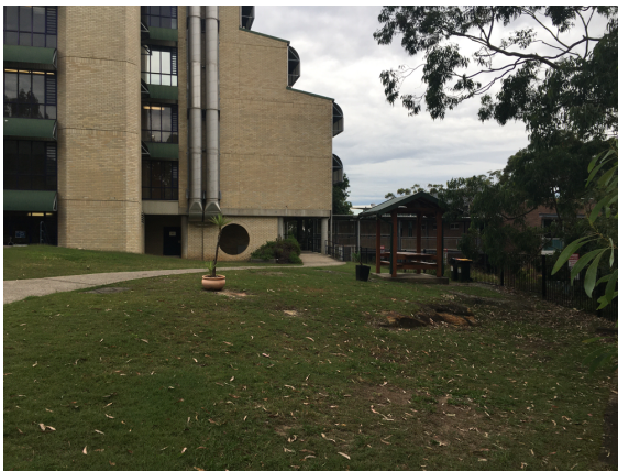
Figure 5.7 View from the north east corner of the proposed carpark with northern aspect of building J.
