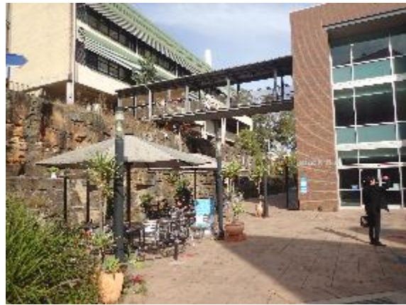
Figure 5.2 Walkway through the sandstone cliff and building K. Note the bridge over the walkway connecting buildings J and K.
