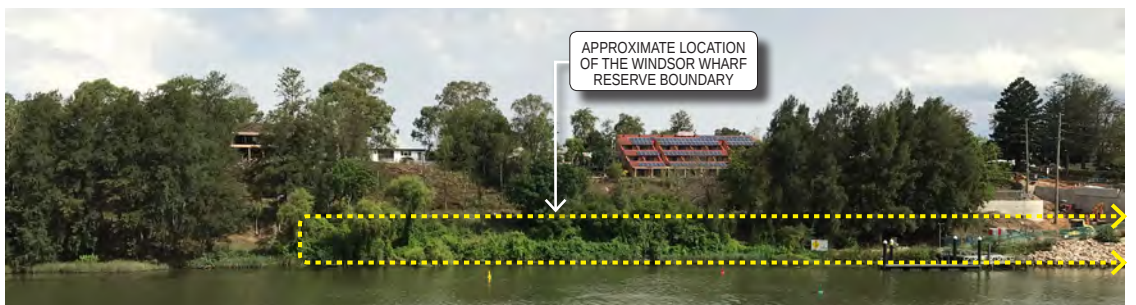
Figure 9. Photographs showing current conditions of the Windsor Wharf Reserve downstream of the Windsor Bridge Replacement project site (smm 12/01/2020)
