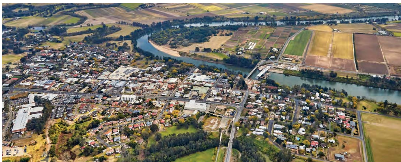
Aerial view of the Windsor Bridge replacement project
