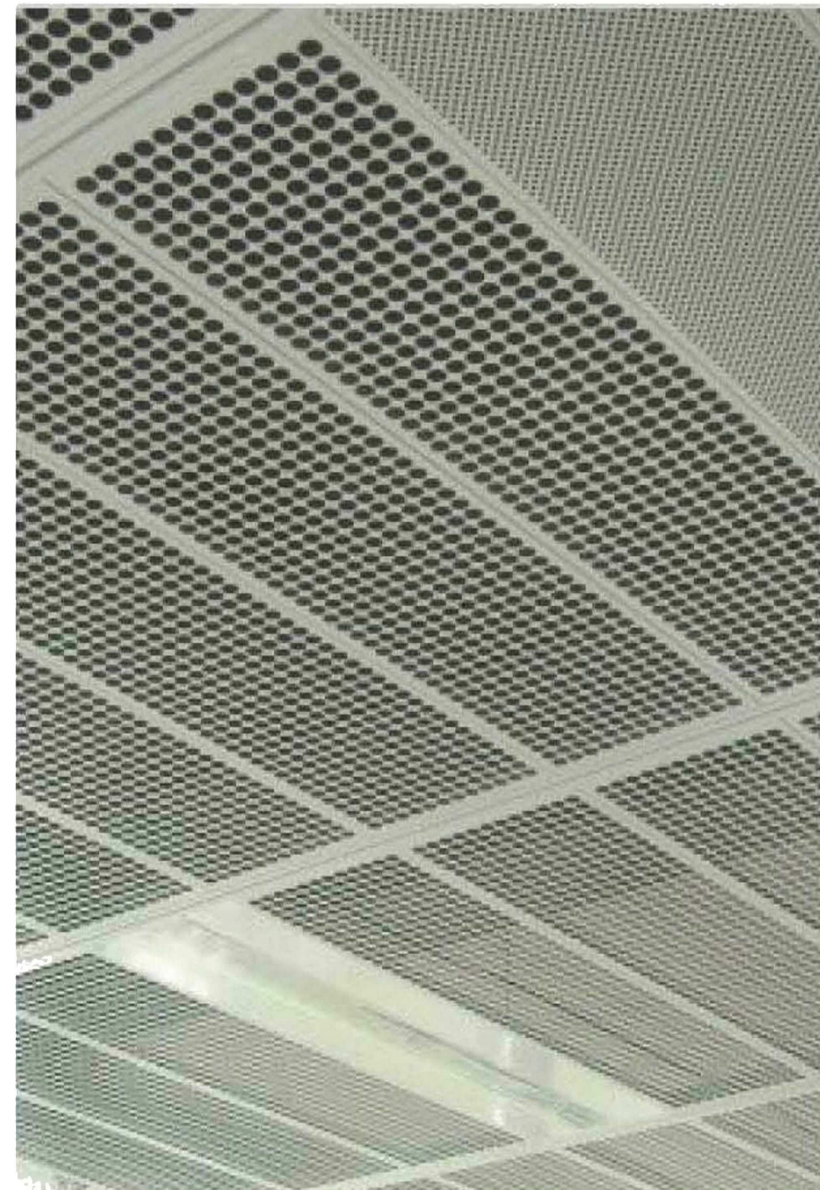
METAL PAN CEILING TO MAKER SPACES
