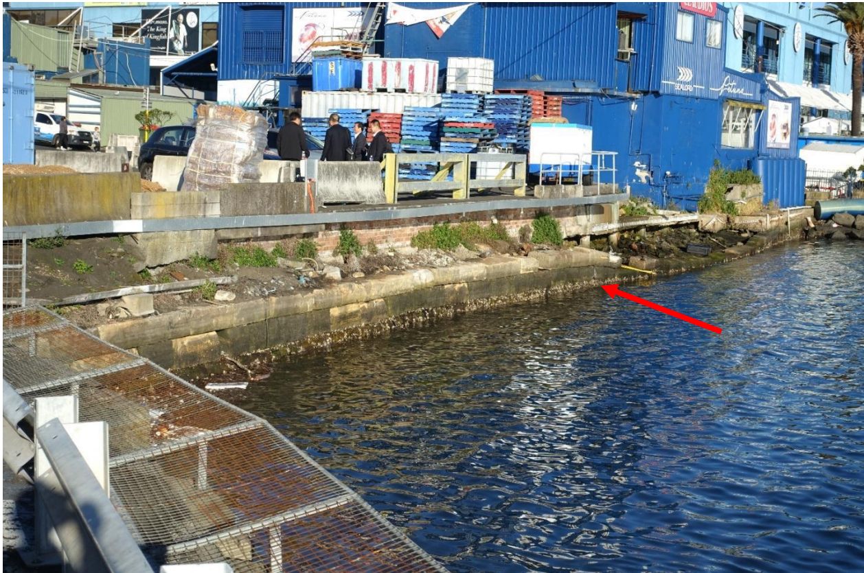
Figure 15: Where the existing sandstone seawall terminates (red arrow) may mark the entrance to the c.1880s dry dock/ slipway.
