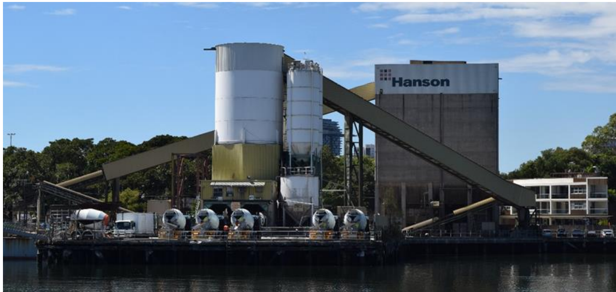
Figure 18: The Hanson Heidelberg cement concrete batching plant.
