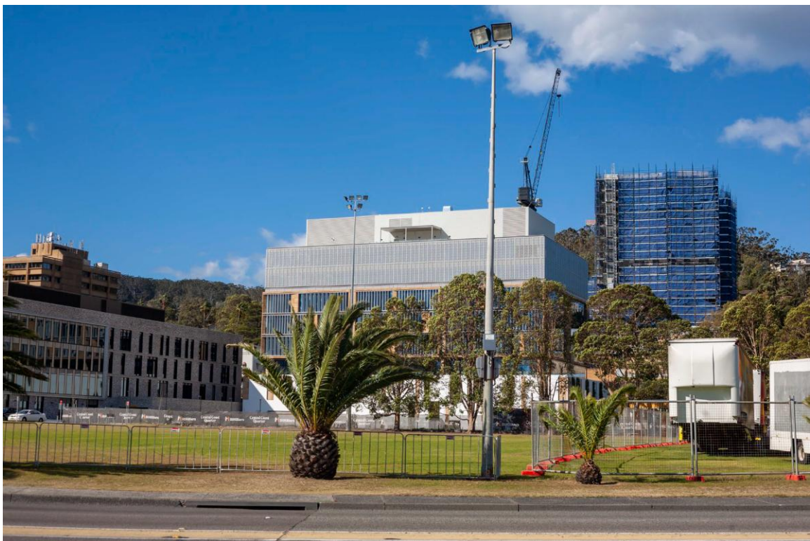
Figure A16. A current view from the waterfront across Central Coast Highway and Leagues Club Fields towards existing building on 26 Mann Street site with palm trees in the foreground & semi-mature Eucalypts along Baker Street in the mid-distance
