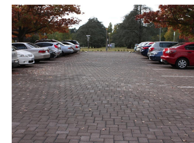
Permeable paver Similar to Hydroston H80, colour to match existing.
