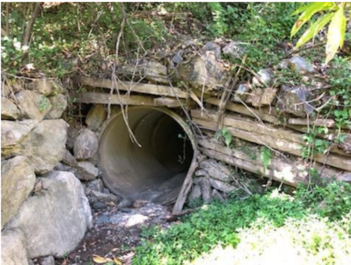
Plate 3 Headwall with timber and argillite rubble/blocks, note the new modern pipe has been extended to be flush with the headwall. Photo facing south east.
