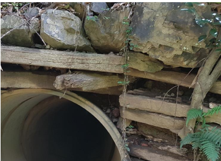
Plate 4 Close up of timber planks and irregular argillite rubble, note the new modern pipe has been extended to be flush with the headwall. Photo facing south east.
