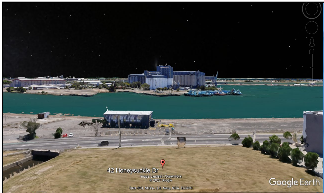
Photo 1 – Google Earth Image from 42 Honeysuckle Drive.
