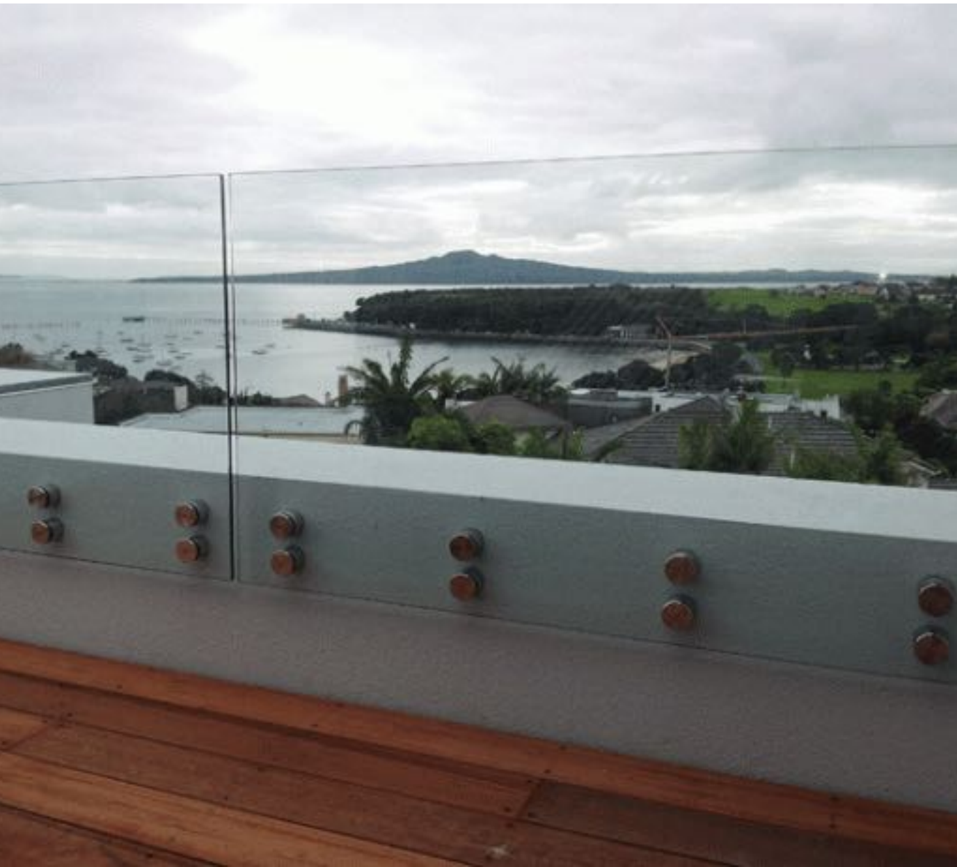
BAL(1) - Frameless glass balustrade fixed to back of white concrete precast upstand (PC) - Northern and South Balconies
