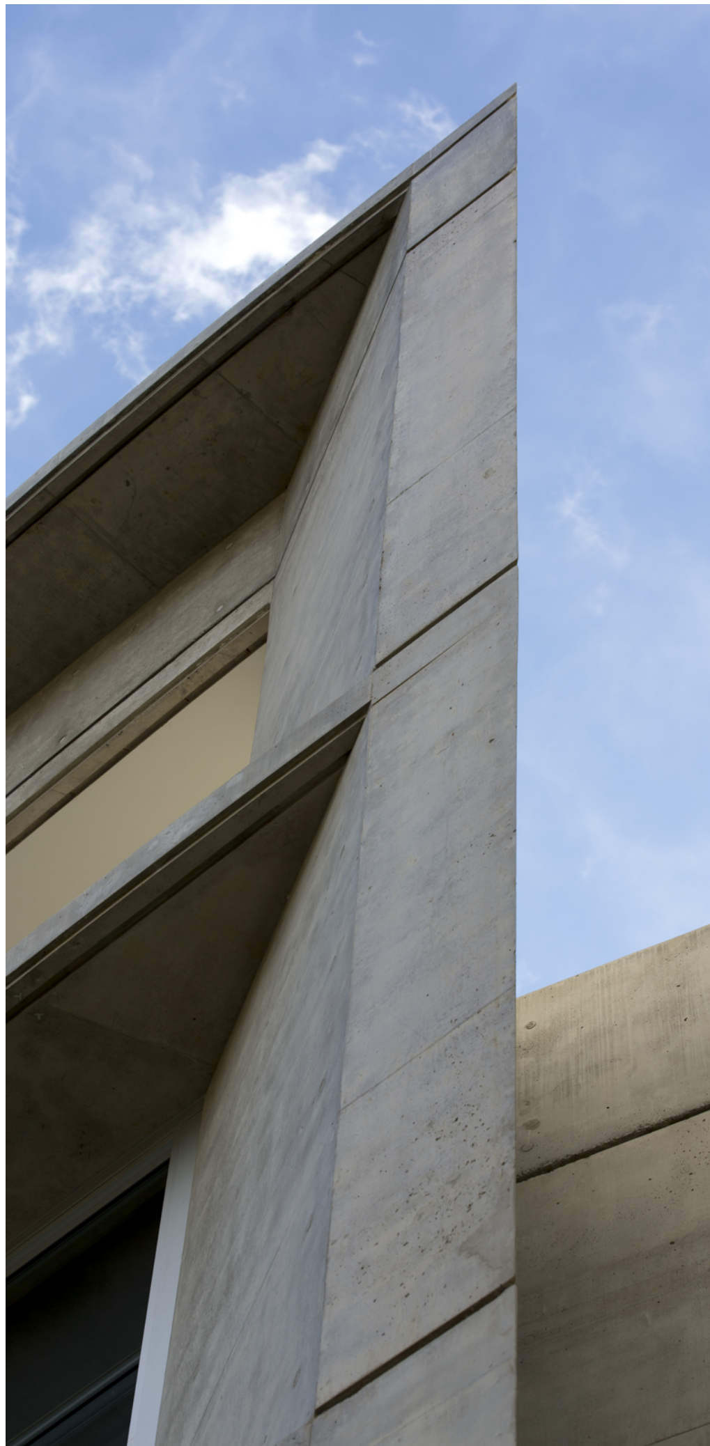
OFC - Class 2 Concrete columns and expressed slabs
