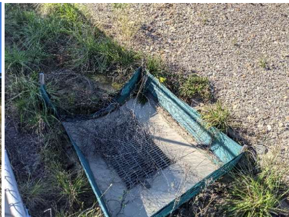
Figure 4 – Inlet pit within swale
