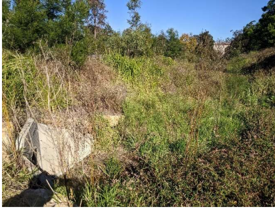
Figure 5 – Headwall Outlet to Swale upstream Basin
