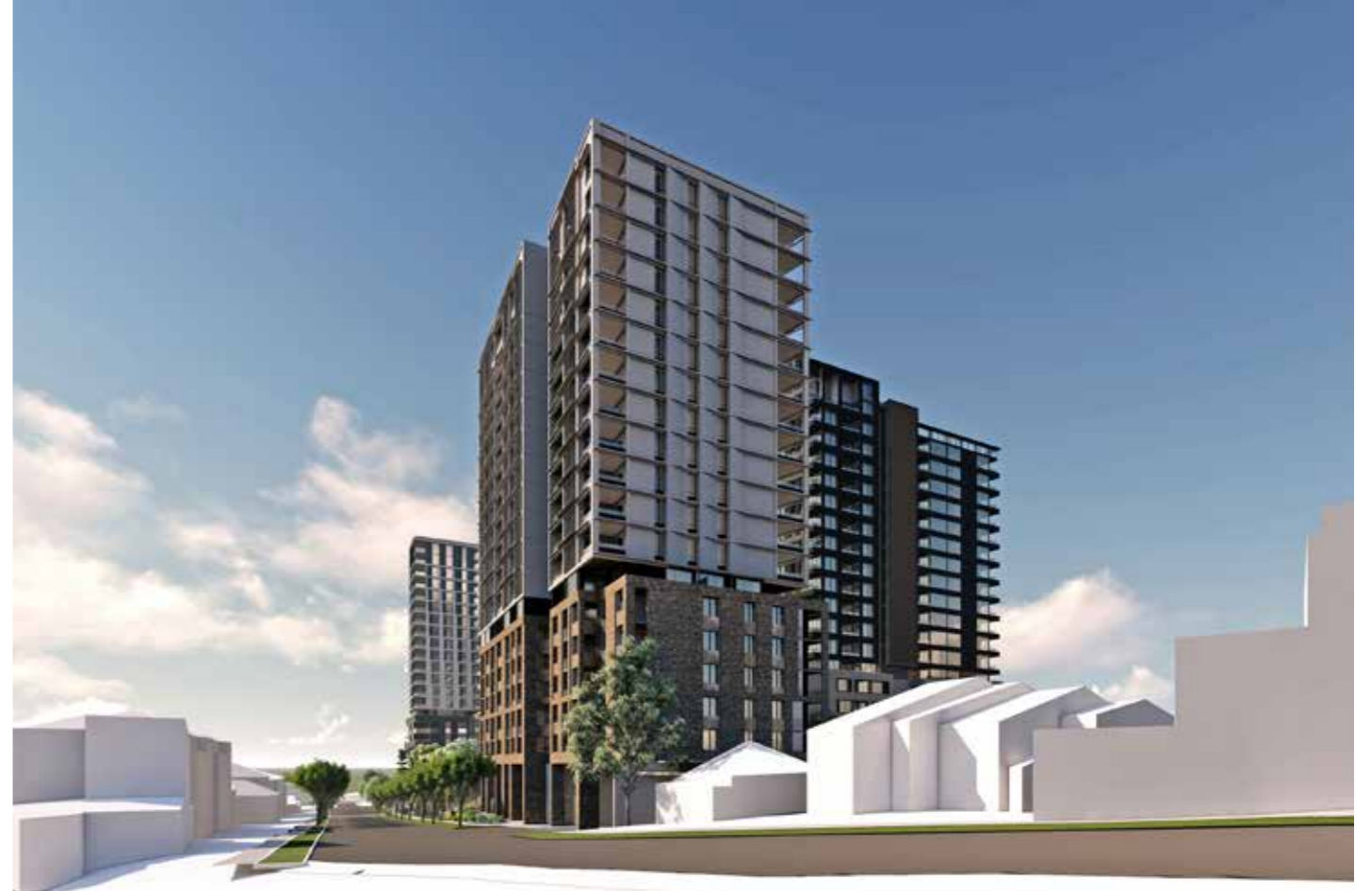
View from south-western corner of site on Eden St
