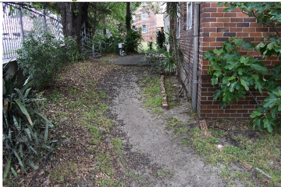
Figure 22: Erosion as a result of water runoff. View looking south
