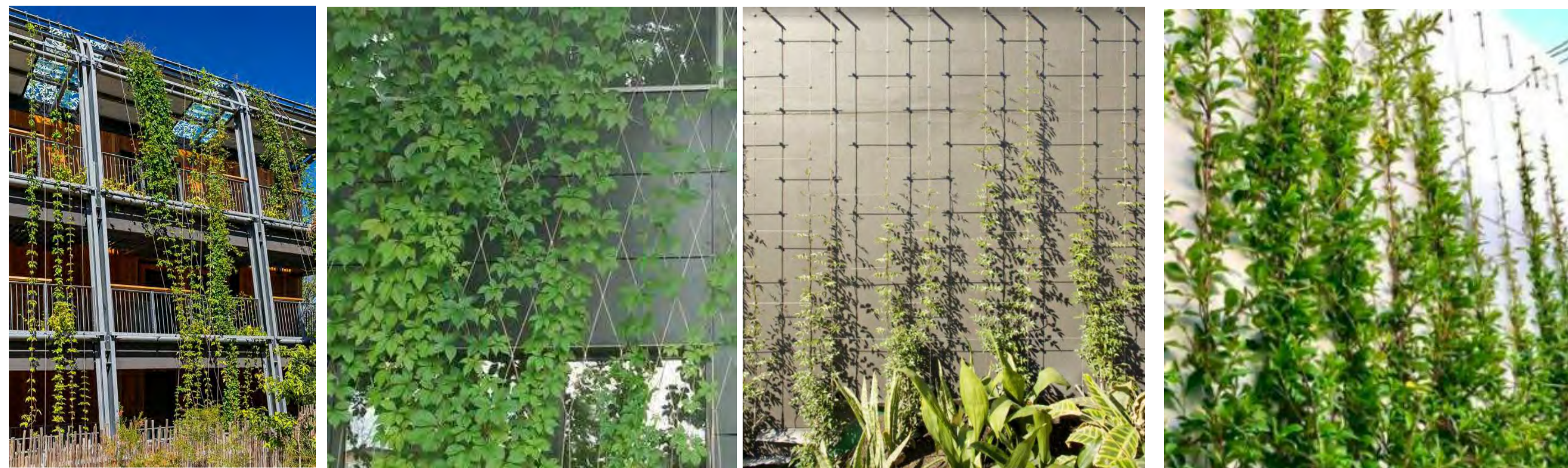
01 STAINLESS STEEL CABLE WIRE GREEN SCREEN [stainless steel wires to support landscape vines on southern side of building]
