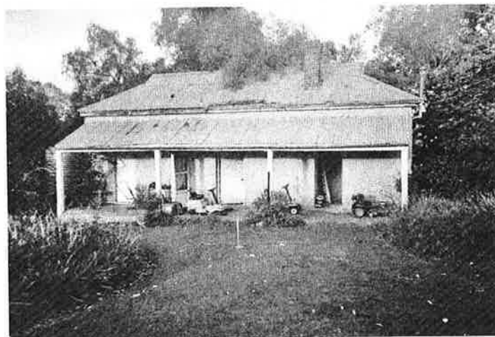
Front elevation of old cottage
