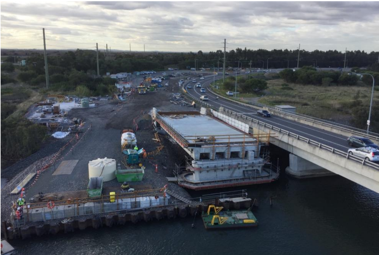
Photo 5-2 Example of a temporary wharf
