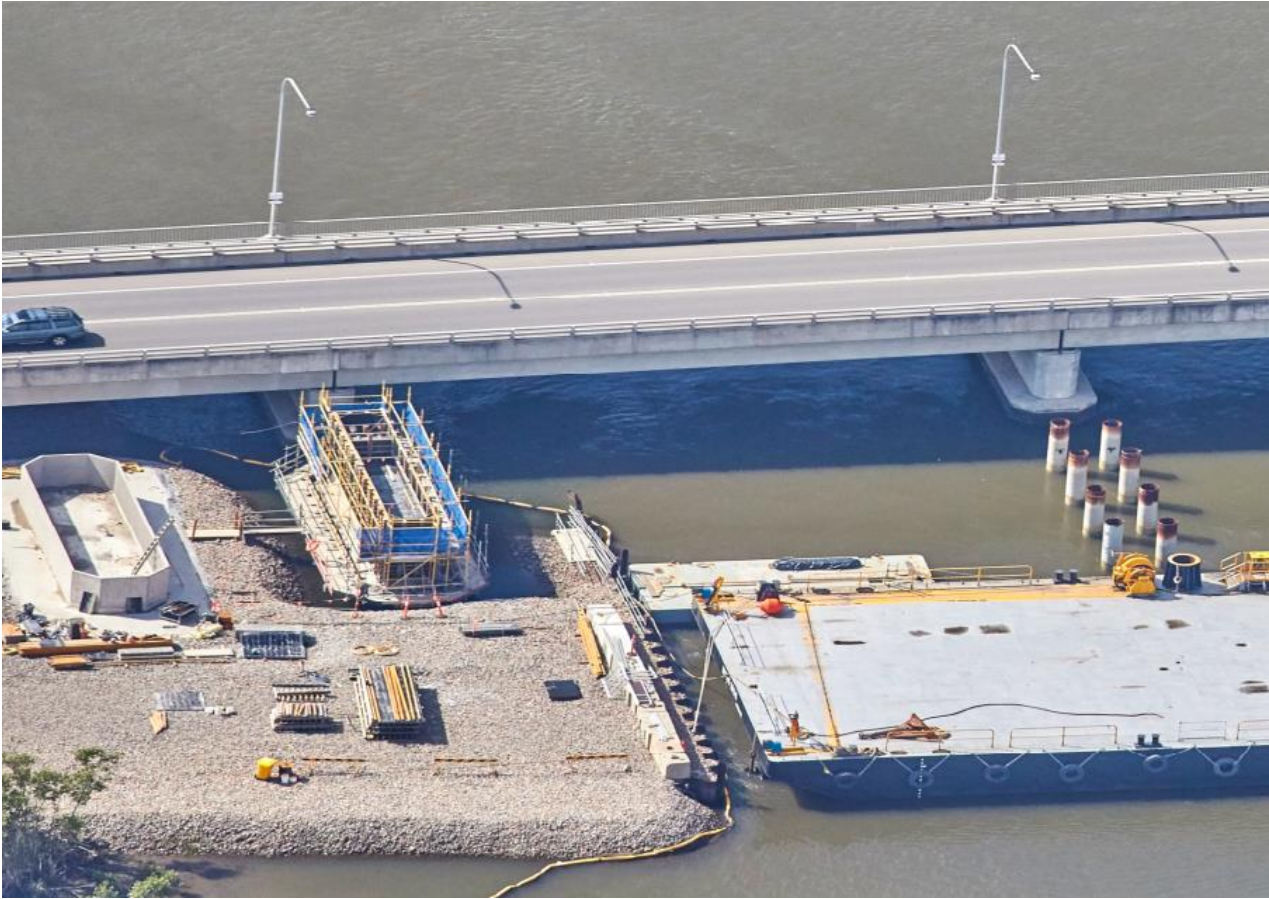
Photo 5-1 Example of a temporary rock platform within a river
