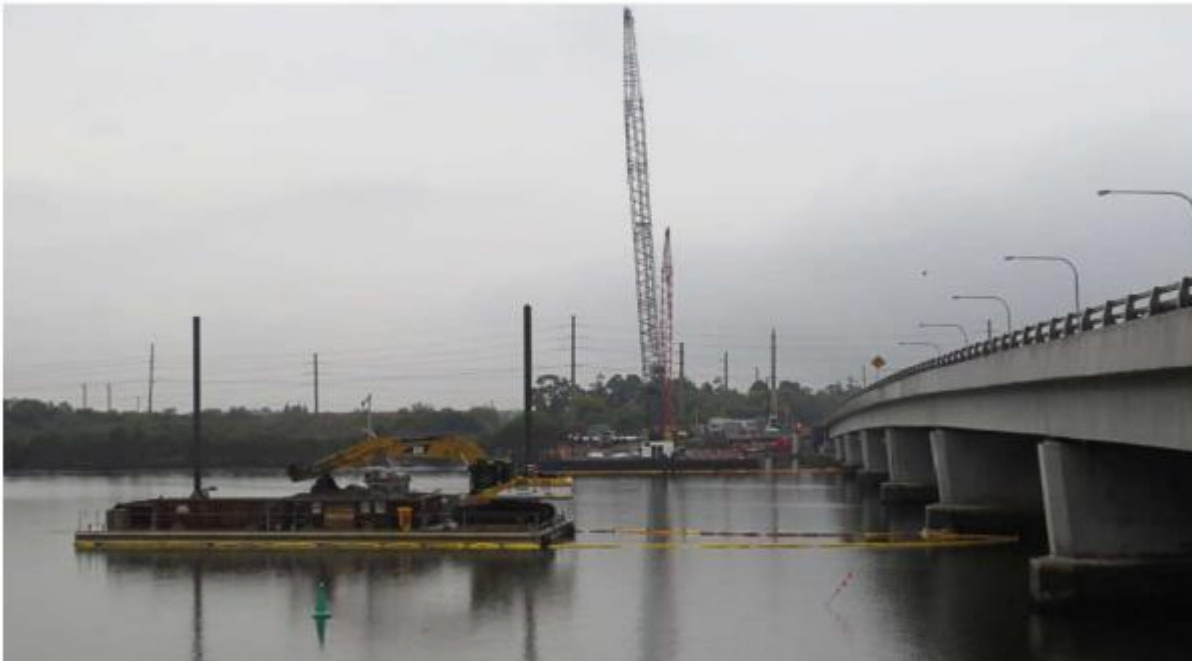
Photo 5-3 Example of dredging the Hunter River
