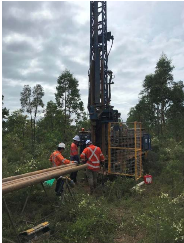
Photo 1 - Typical drill rig setup during augering (BH01)
