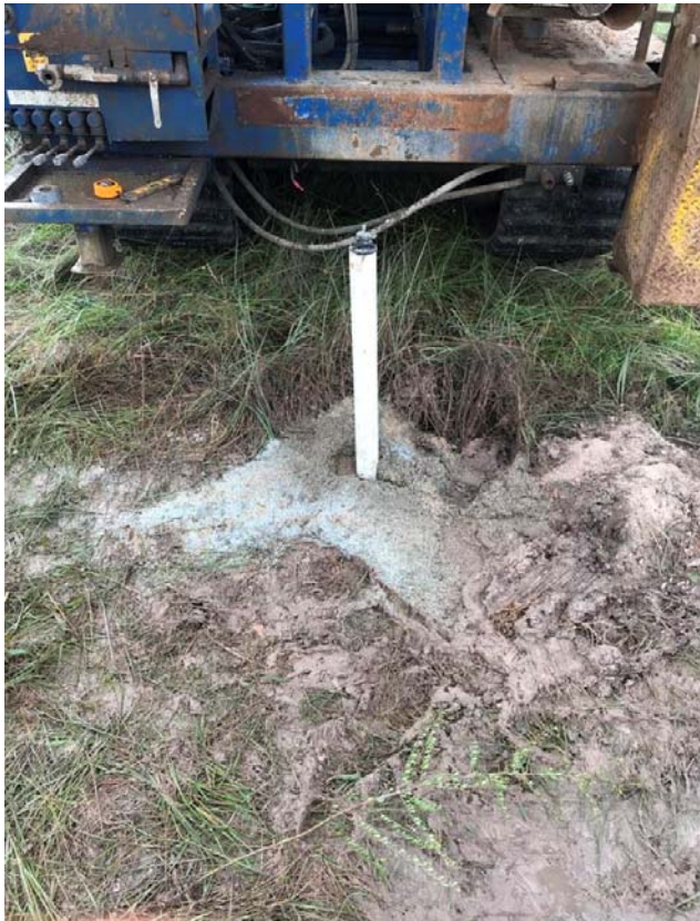
Photo 2 - Typical Standpipe piezometer (monitoring well) setup (BH03)
