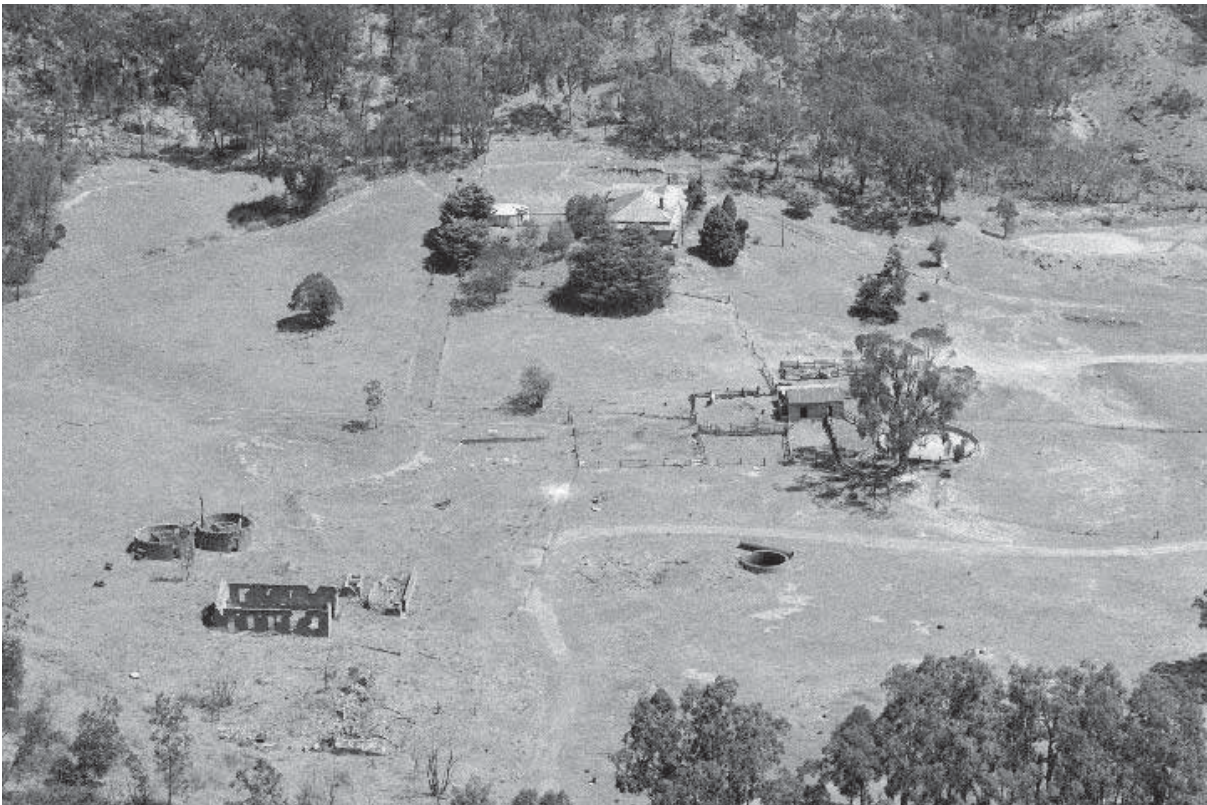
Figure 9: Remains of the Torbane Refinery and transport terminal. The Works Managers House at centre is now privately owned and occupied. (Source: Ayling, B op cit)
