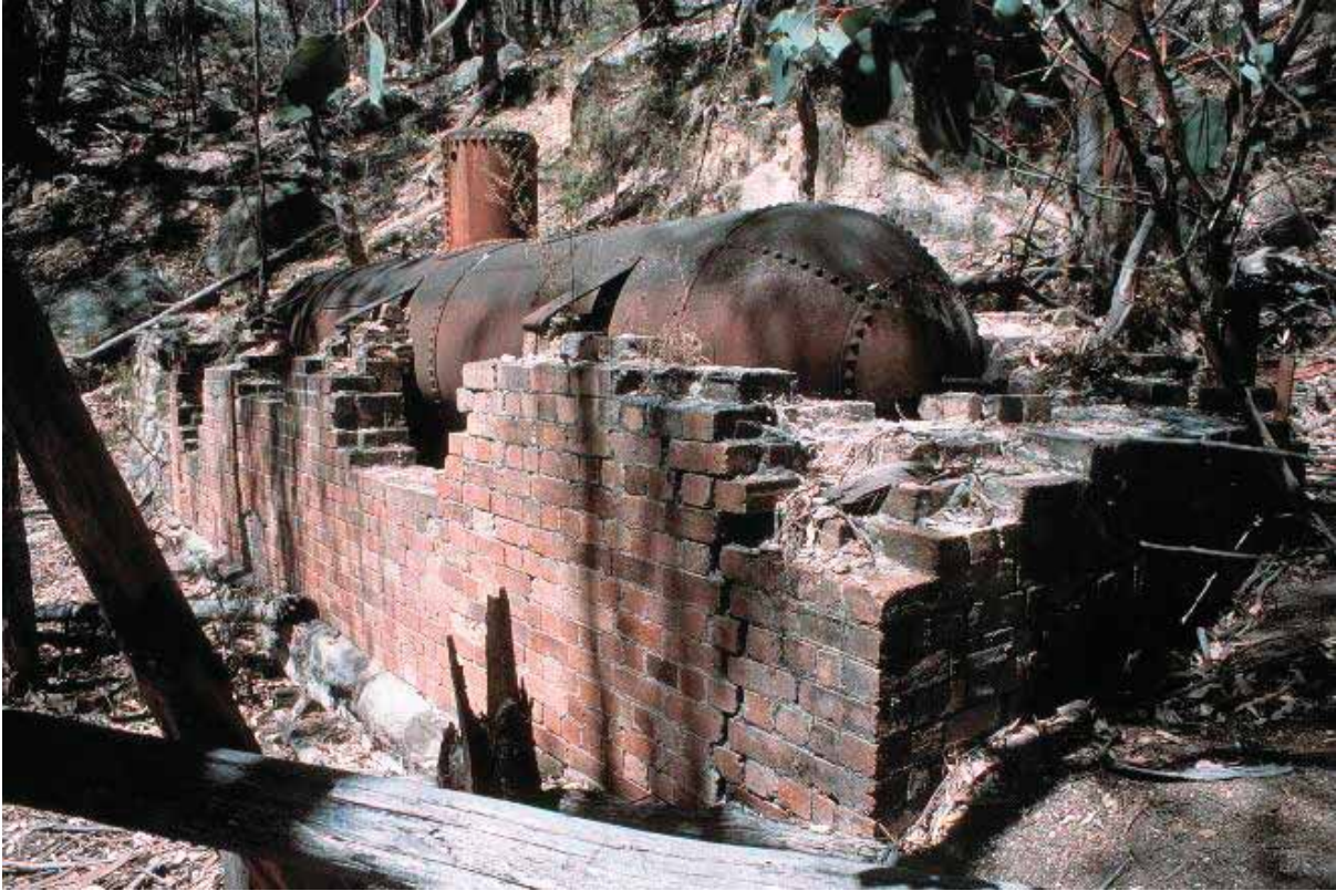
Figure 8: Egg-end boiler associated with the Cable tramway haulage system (Source: Ayling, B op cit)
