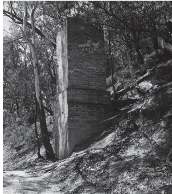
Figure 11: Mine Ventilation Chimney (Source: Ayling, B op cit)
