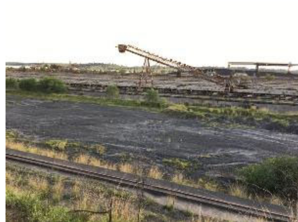
Photo 5-15: The coal stockpile areas near Liddell. This large area contains concrete and gravel surfaces with regrowth weeds.
