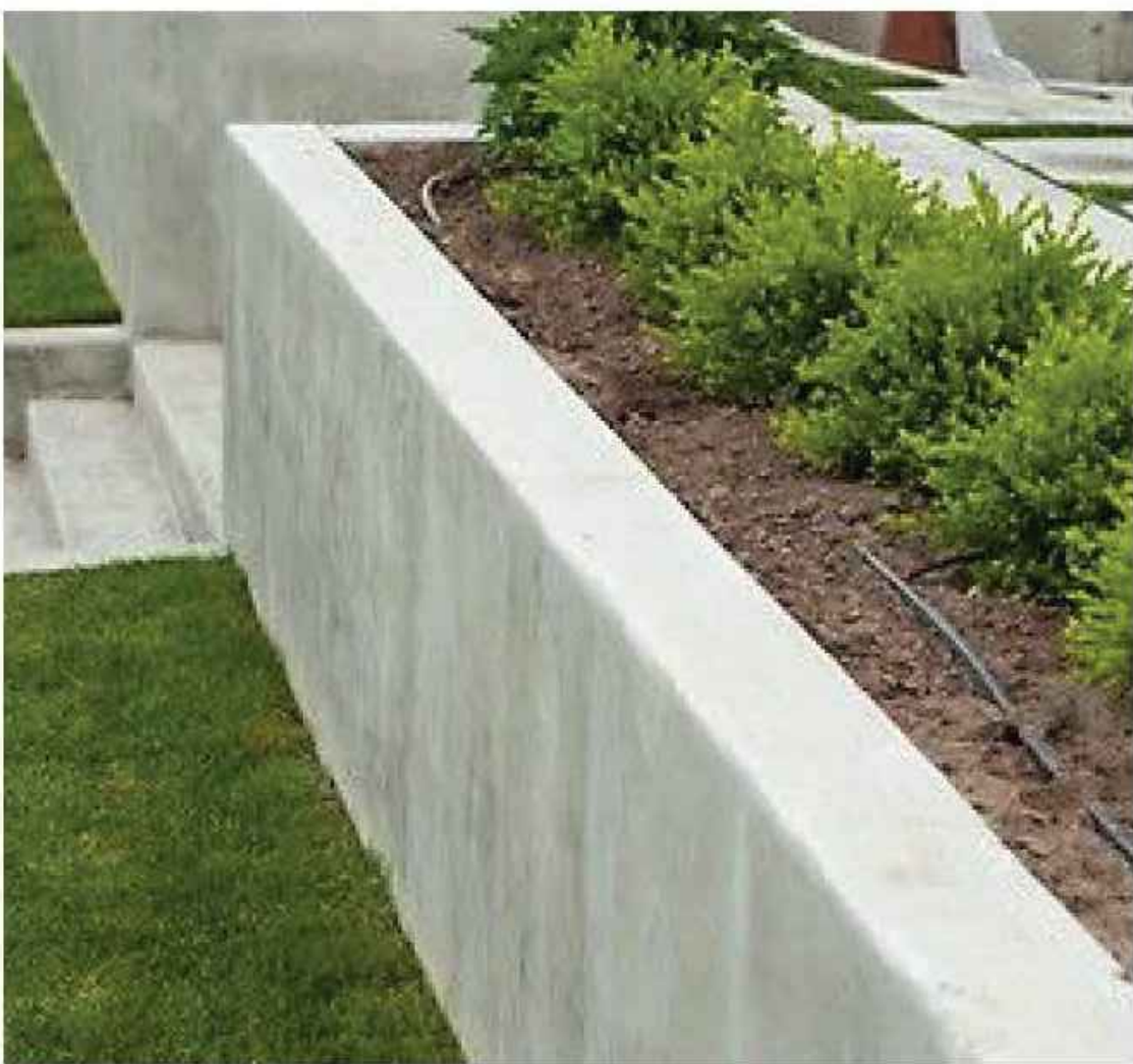
In-situ concrete walls
