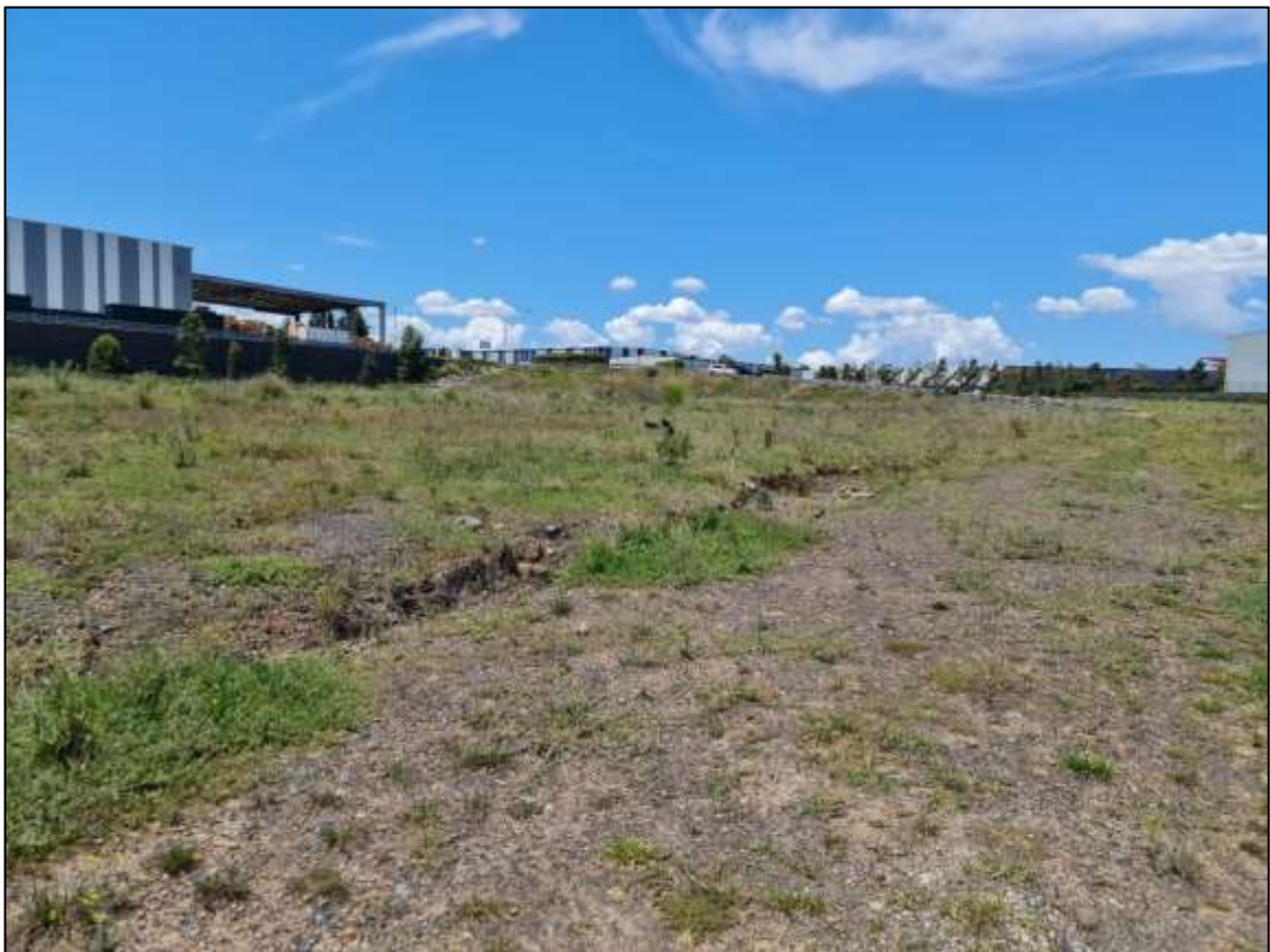
Figure 4.1 Project area looking back to the entrance from the south-west corner, note erosion rill through the fill
