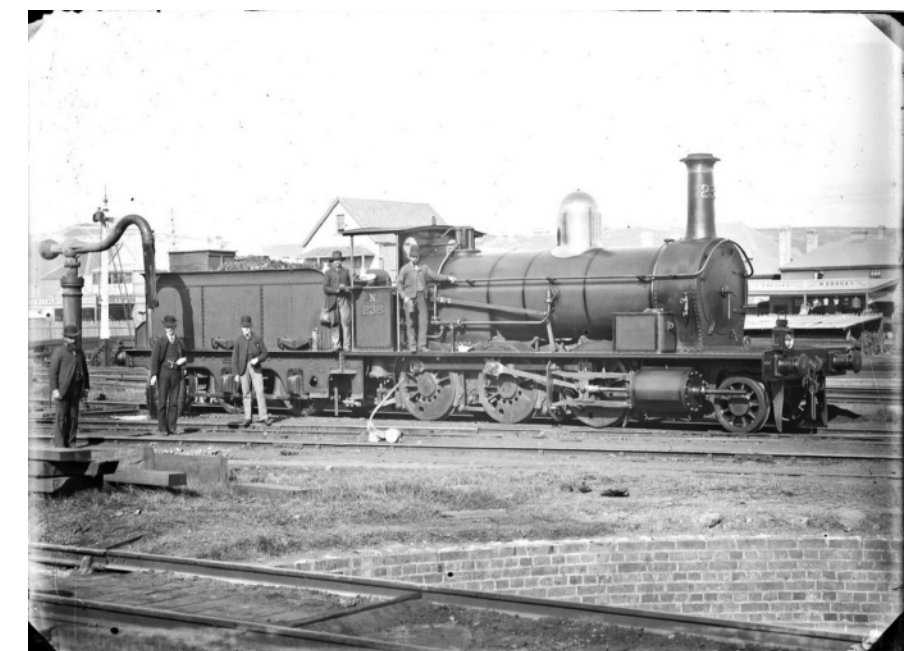
Locomotive and Turntable at Honeysuckle, installed 1857
