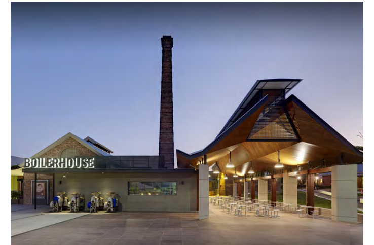
Boilerhouse heritage adaptation, WSU Rydalmere
