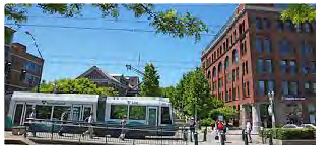
Figure 2.1.2: University of Washington Tacoma, Light Rail Station
