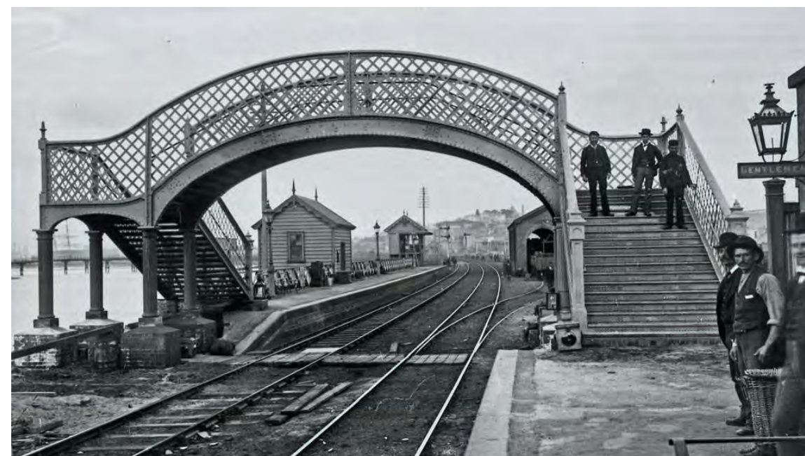
Honeysuckle Station on the waterfront, built 1872
