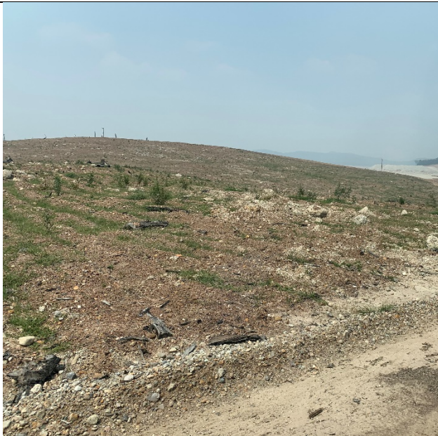
Plate 3: Areas reshaped, topsoiled and seeded with logs and sticks placed across the landform as habitat features (standing trees in background).
