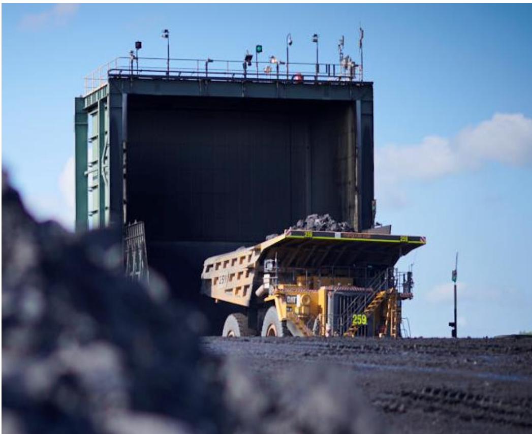
Plate 3.5 Existing ROM Hopper Enclosure at Mangoola Coal Mine
