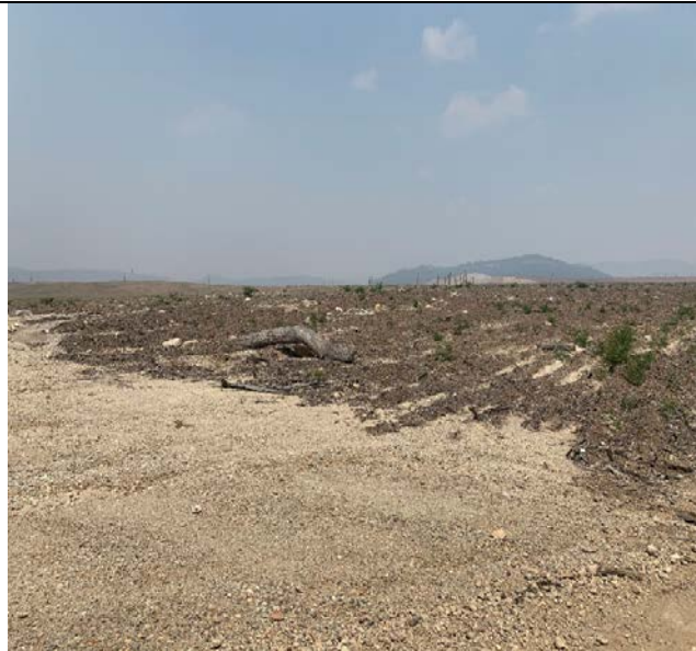
Plate 2: Areas reshaped, topsoiled and seeded with logs and larger sticks placed across the landform as habitat features (standing trees in background).
