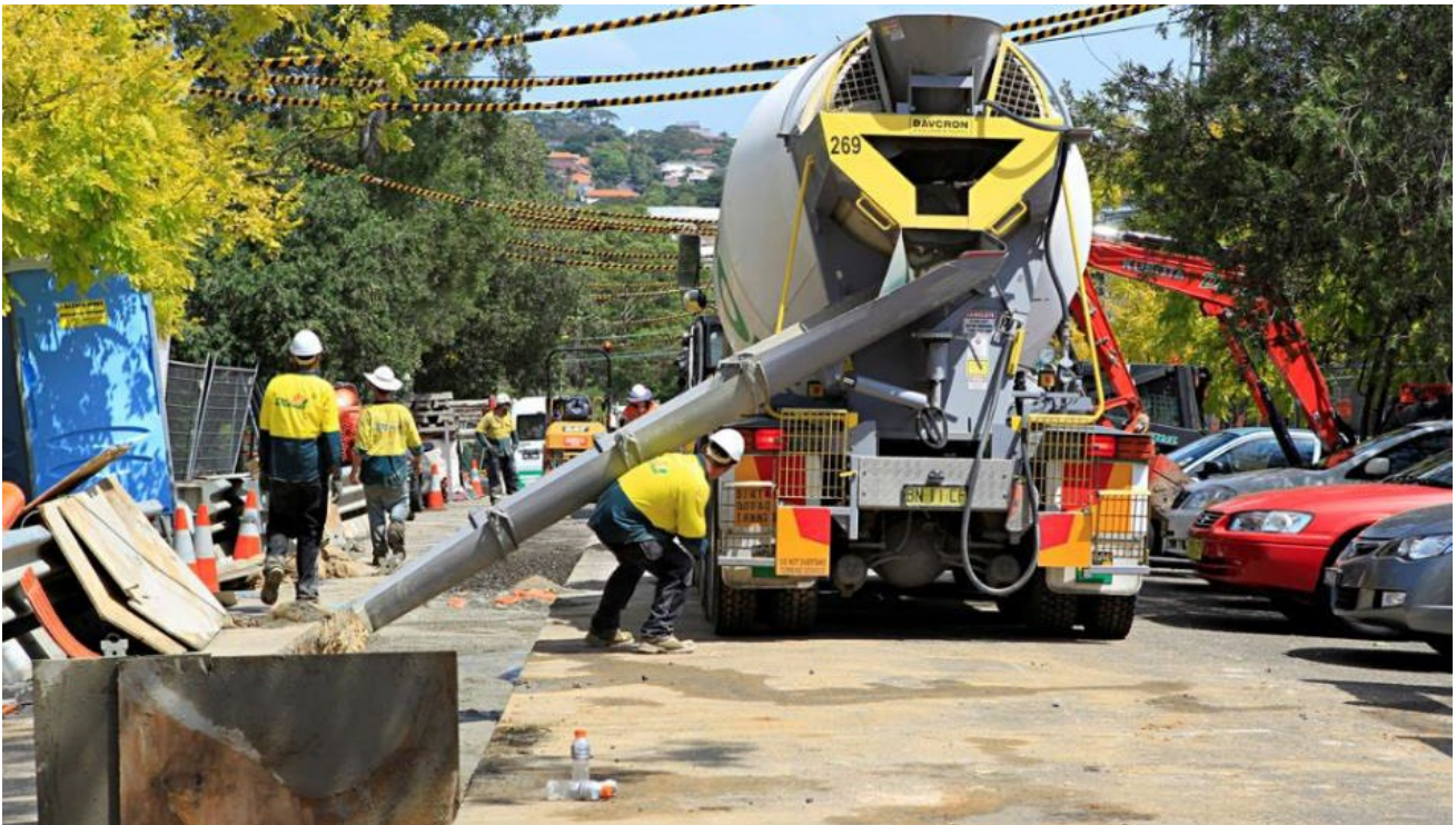
Photograph 8.9 TSB being poured over conduits
