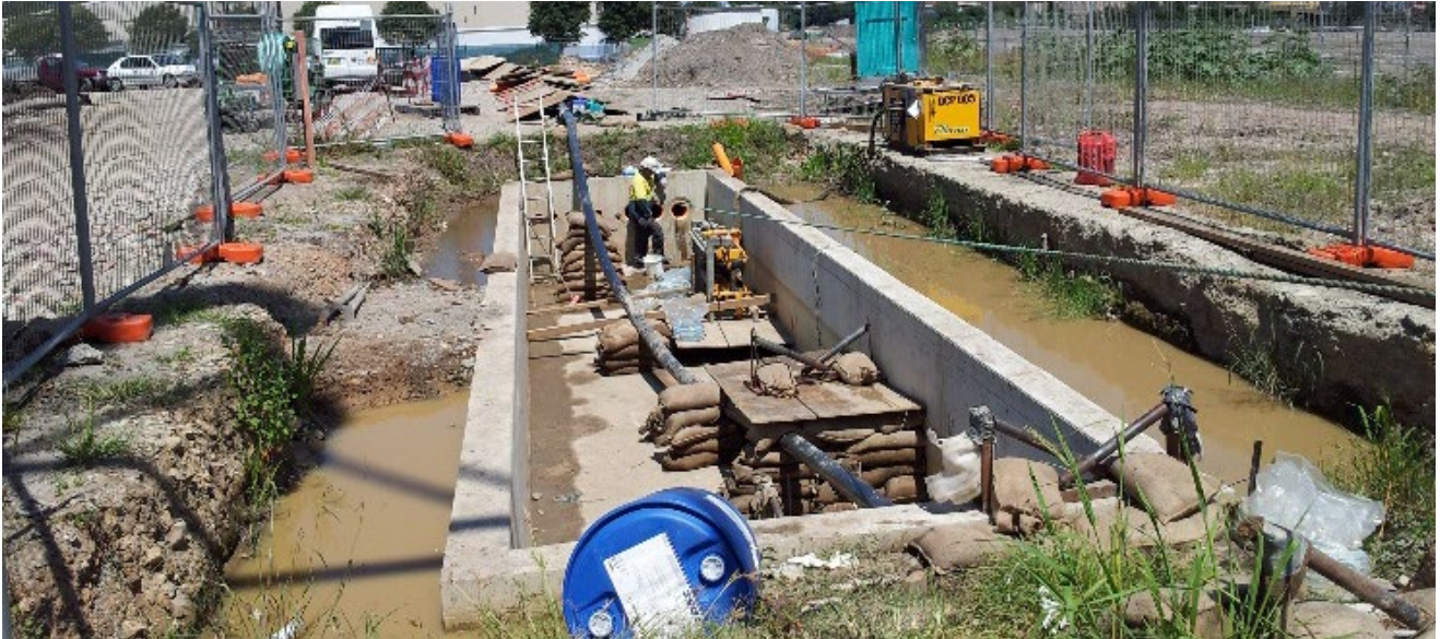
Photograph 8.8 Typical joint bay being installed in Australia
