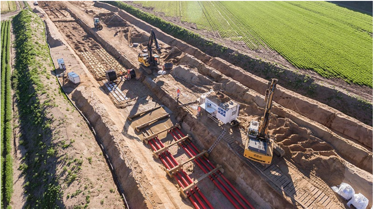
Photograph 4.3 Example of cable installed in a surface trench using a cut and cover excavation method
