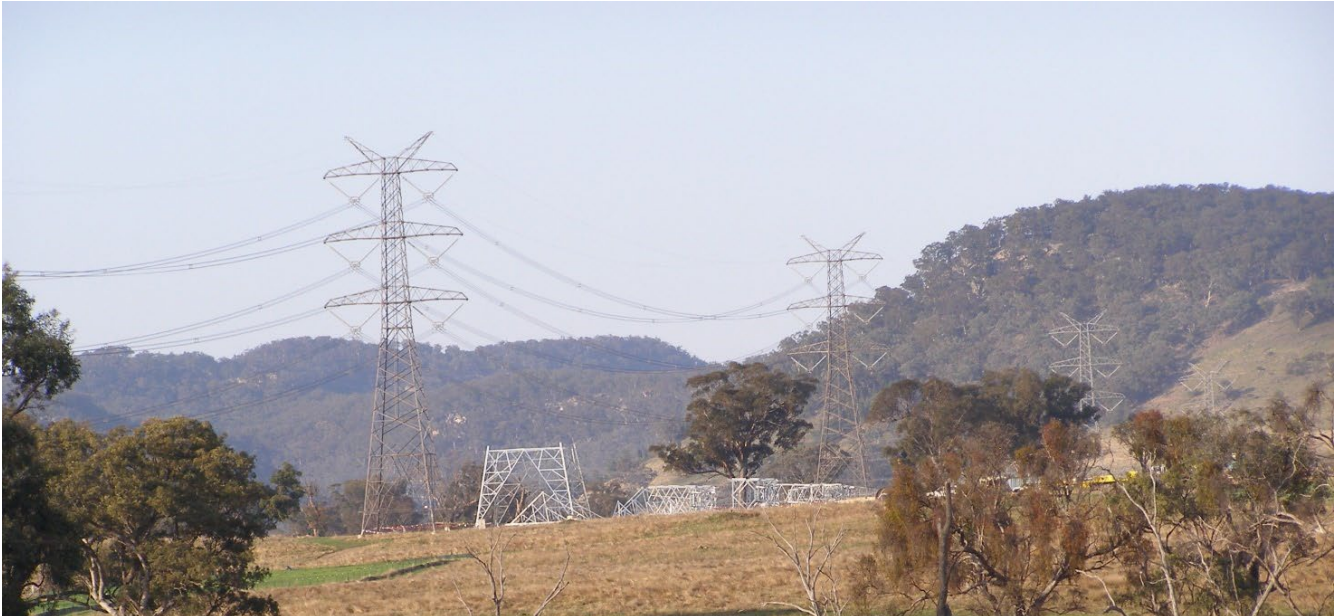
Photo 4-6 Example of the Initial construction of new galvanised structure adjacent to existing structure which has subject to natural environmental ageing
