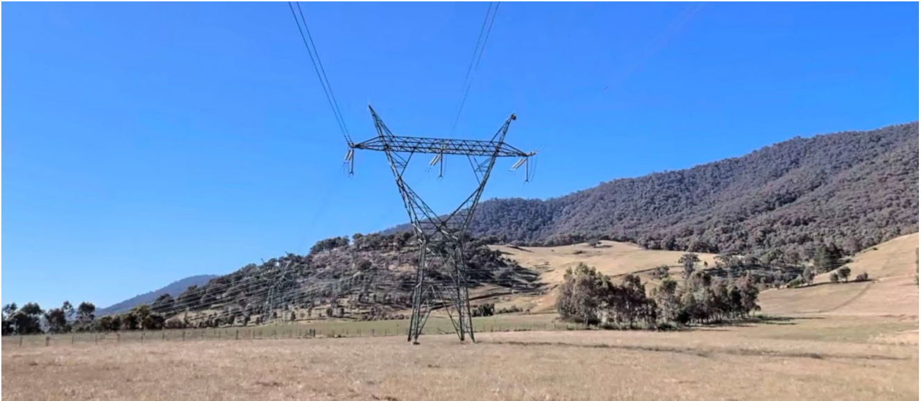
Photo 4-7 An example of painted steel lattice structures
