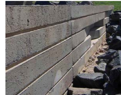
Concrete Retaining walls
