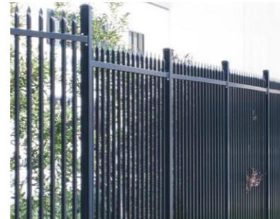
1.8m Security Perimeter Fence
