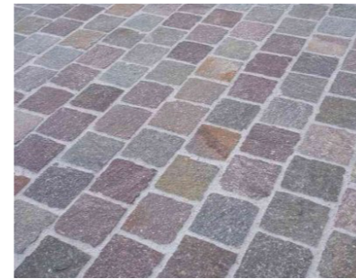
Porphyry Cobblestone Paving
