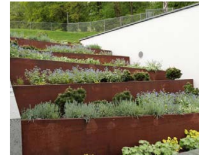
Corten Steel Terracing Retaining Walls
