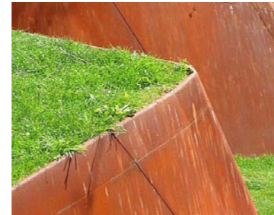
Corten Steel Retaining walls (up to 600mm)
