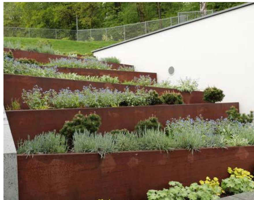
Corten Steel Terracing Retaining Walls
