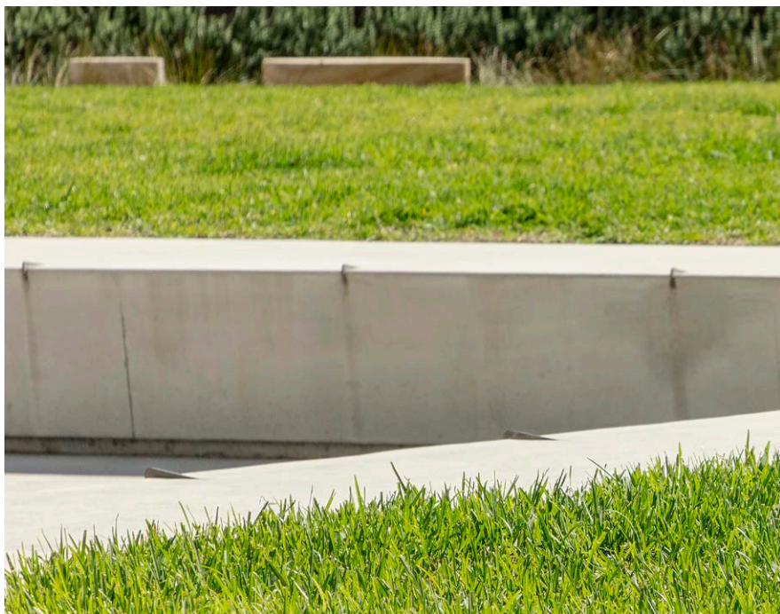
Concrete Retaining walls
