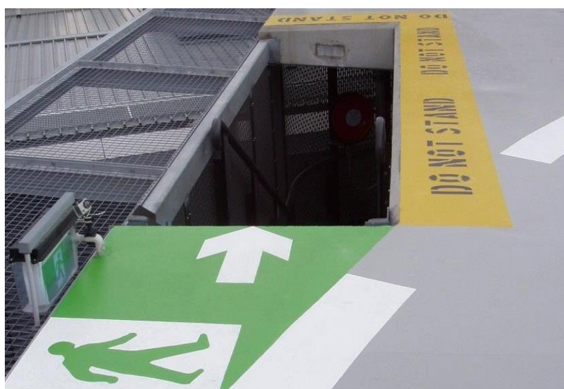
Figure 21: Example of an HLS Deck Emergency Egress Exit
