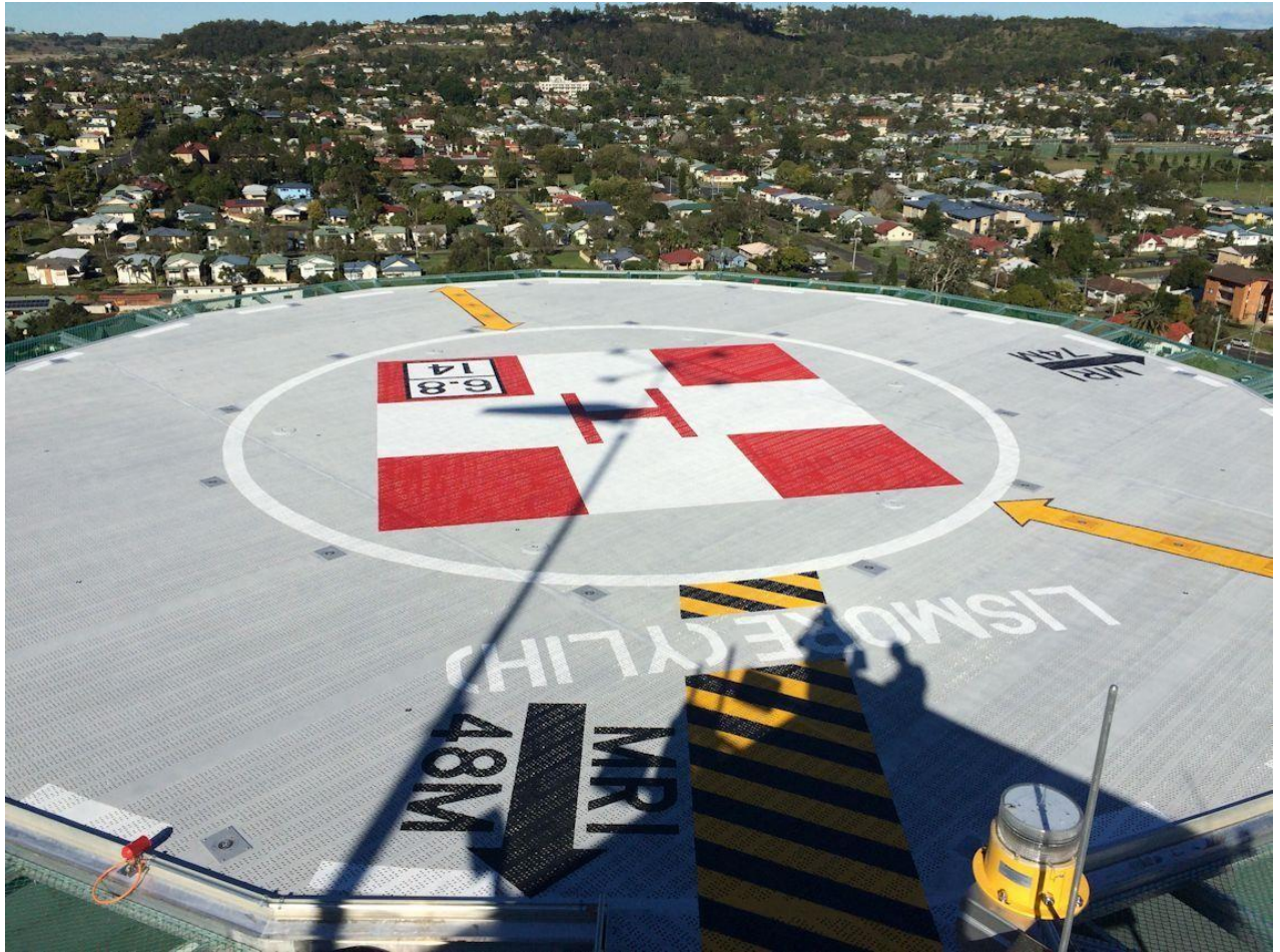
Figure 29: Lismore Hospital Aluminium HLS Deck
