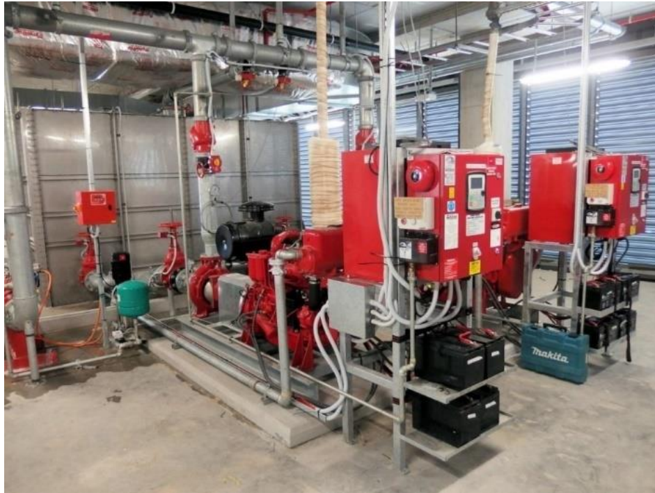
Figure 10: Water DIFFS Storage Tank with Primary and Back-up Pumps
