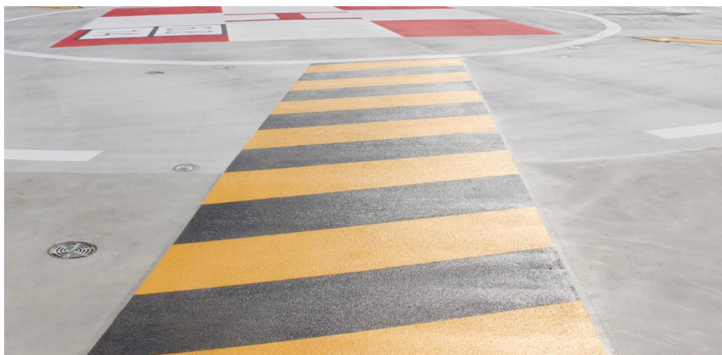
Figure 20: Example of a walkway between the TLOF and the lift vestibule
