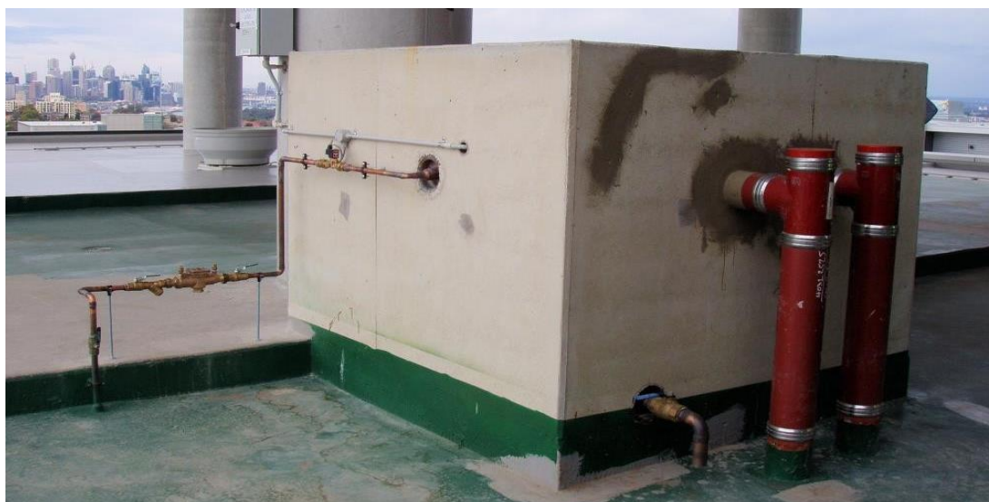
Figure 23: Example Fuel/Water Separator (Puraceptor)
