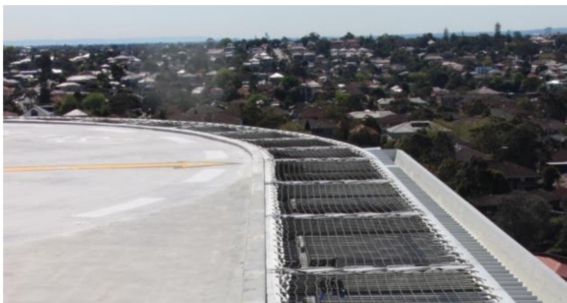
Figure 19: Example of a safety net on a rooftop HLS
