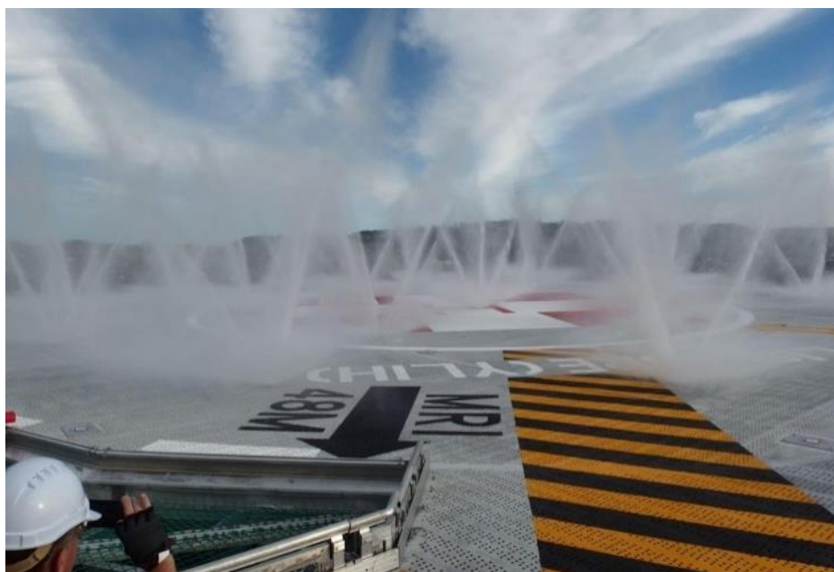
Figure 9: Example of an activated water DIFFS
