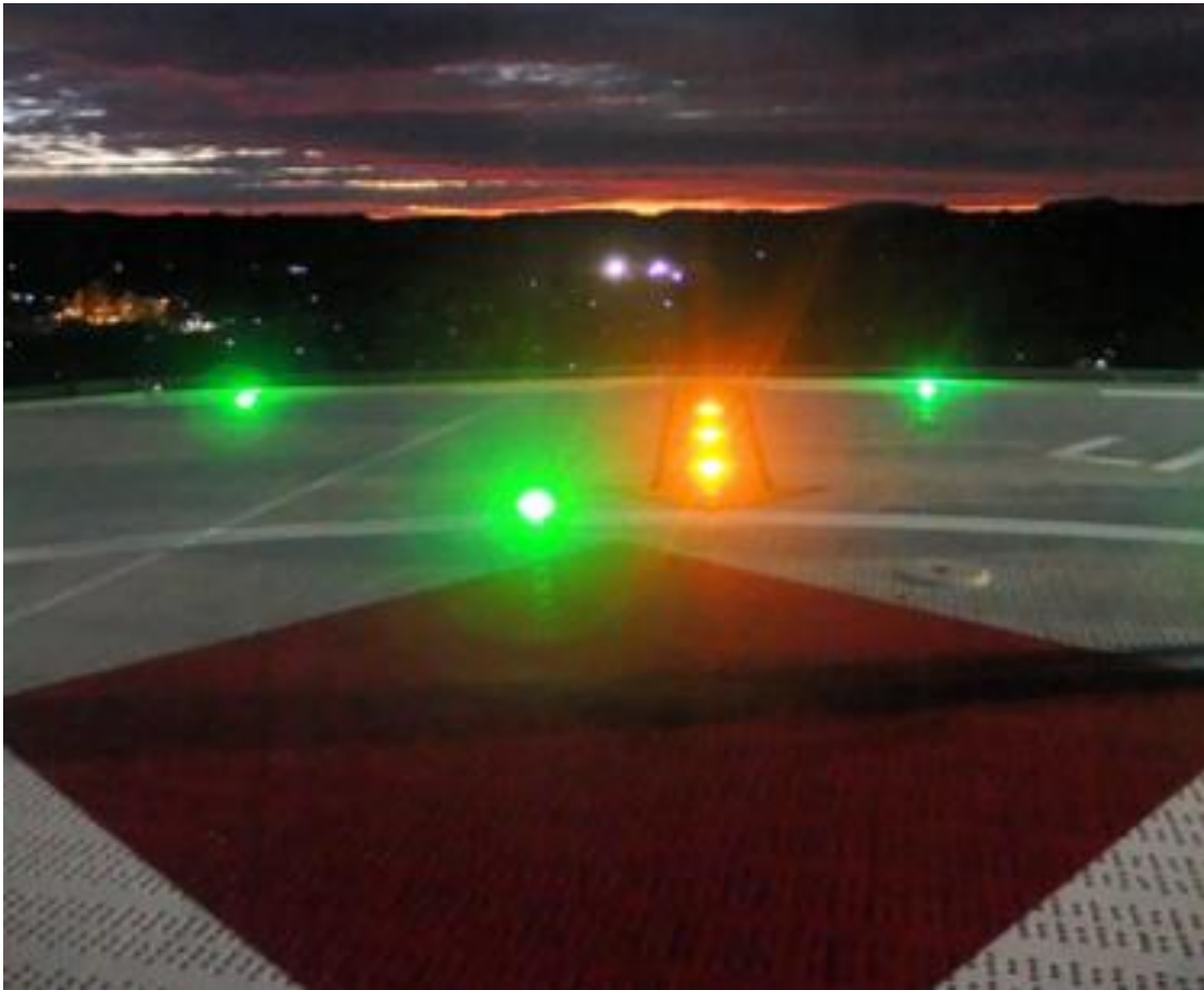
Figure 33: HLS Deck and Approach/Departure Path Lighting Figures 34 shows Lismore Hospital HLS with associated services
