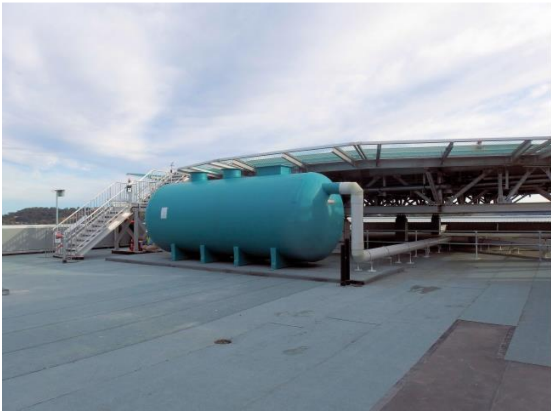
Figure 34: Lismore HLS with 26,150 litre fuel/water separator and escape stairs
