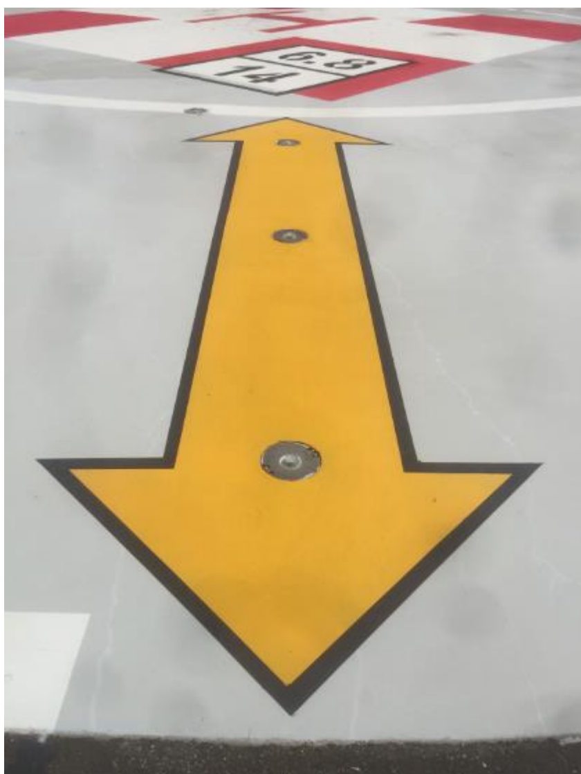
Figure 7: Approach/Departure Directional Arrow and Lights
