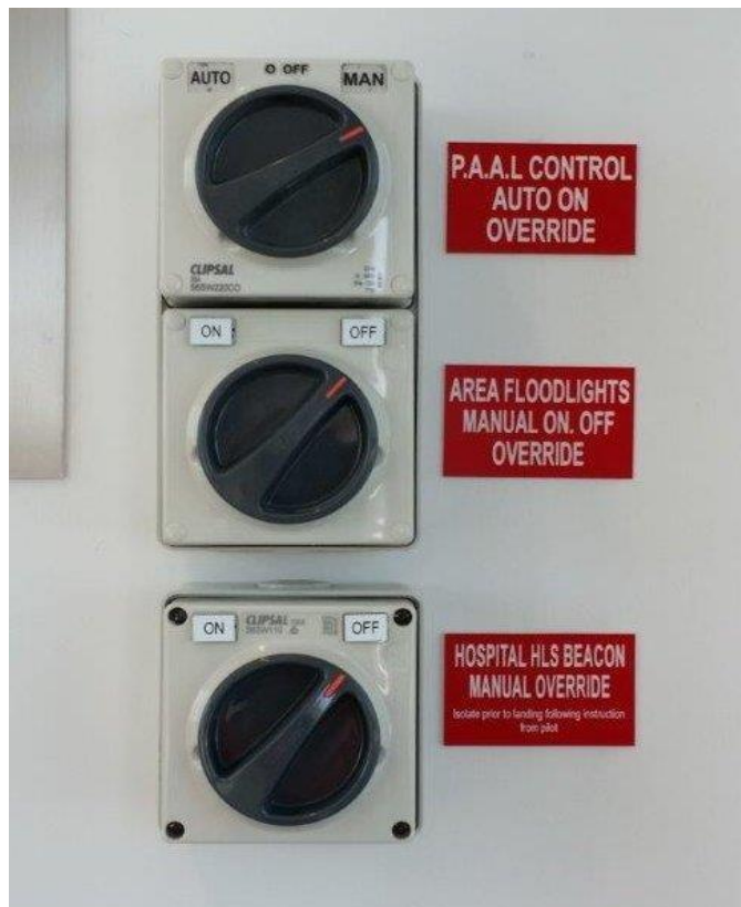
Figure 18: Example HLS Lighting Override Switches
