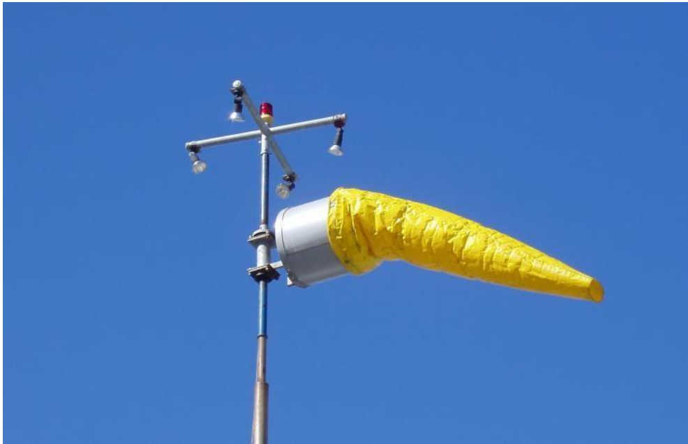
Figure 8: Example Windsock Lighting
