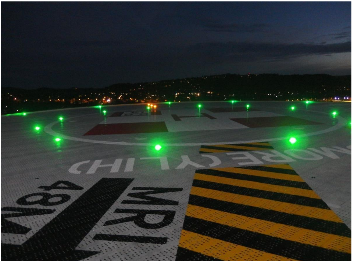
Figure 32: HLS Deck Lighting
