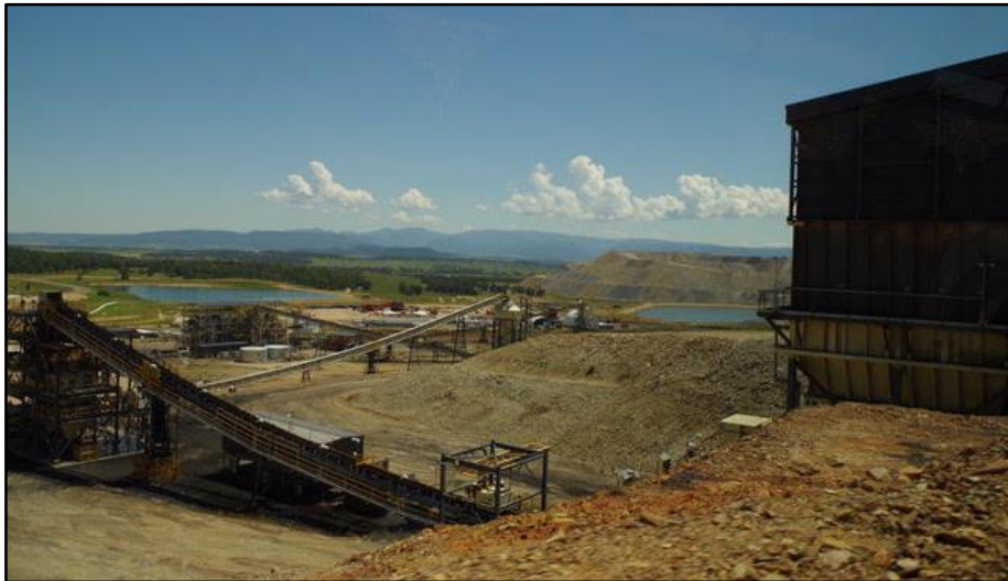
24 hr coal handling and processing plant (CHPP) Maules Creek
