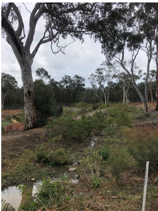
Figure 5 Stormwater diversion drain along north eastern side of leachate dam (north west direction) – stormwater evident in drain due to wet weather condition
