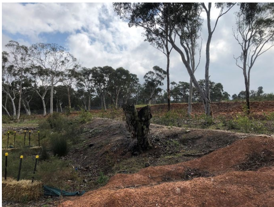
Figure 7 Embankment to stop leachate overflow
