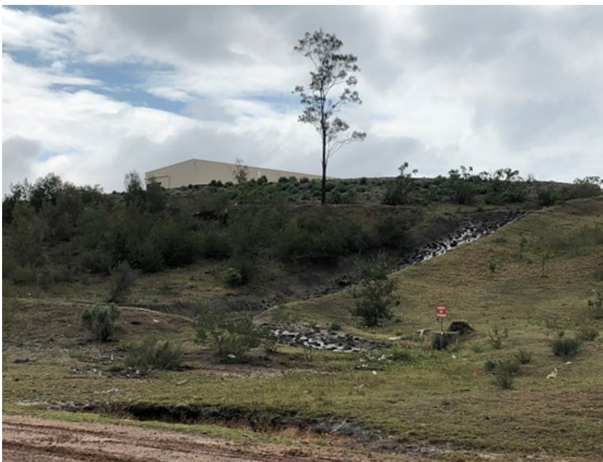
Figure 10 Slope Channel with in-built rocks to reduce speed of run off from Stage 1 – north east direction
