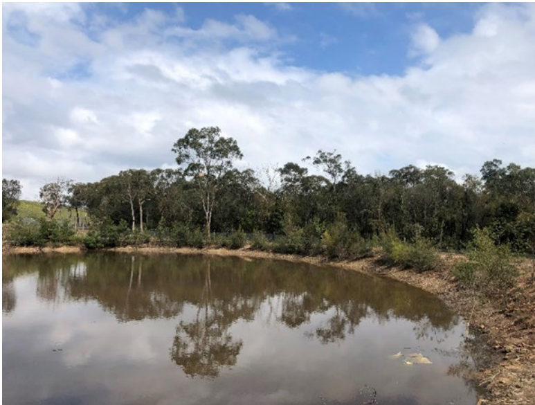
Figure 3 Leachate Dam showing earth embankment – west direction
