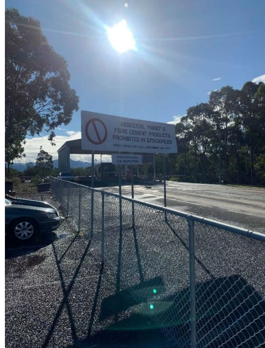
Plate 7 – Weighbridge Cover & Prohibition Sign
