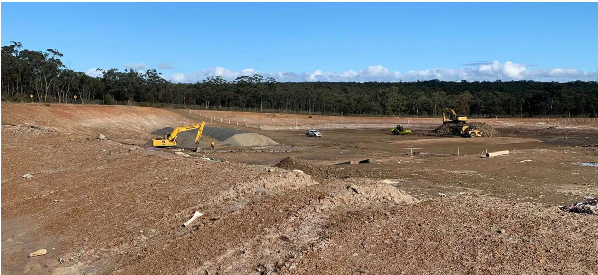
Plate 28 – Future Landfill Cell Preparation
