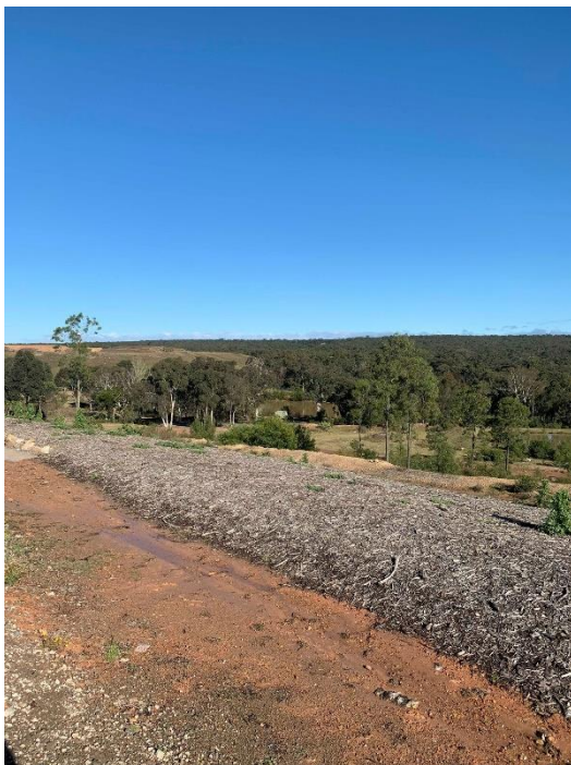
Plate 18 – Stormwater Drain Top of Batter (2)
