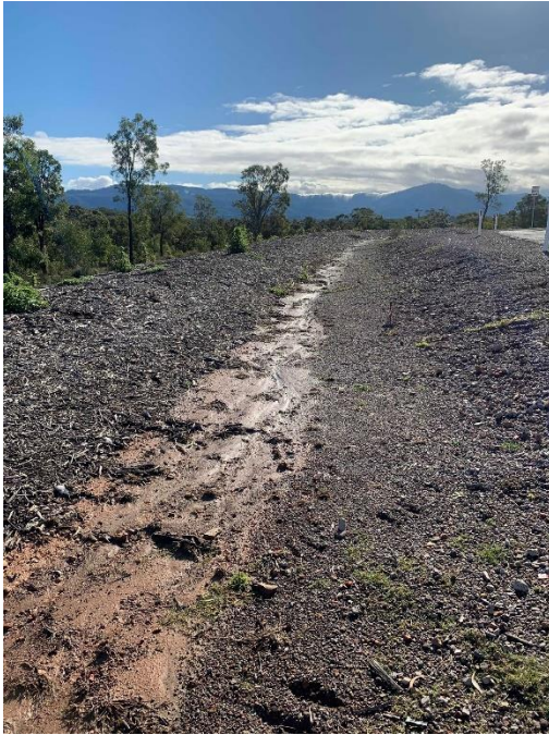
Plate 17 – Stormwater Drain Top of Batter (1)
