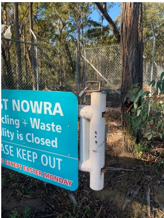
Plate 2 – Site Entry [Gate Lock / Security Fence]
