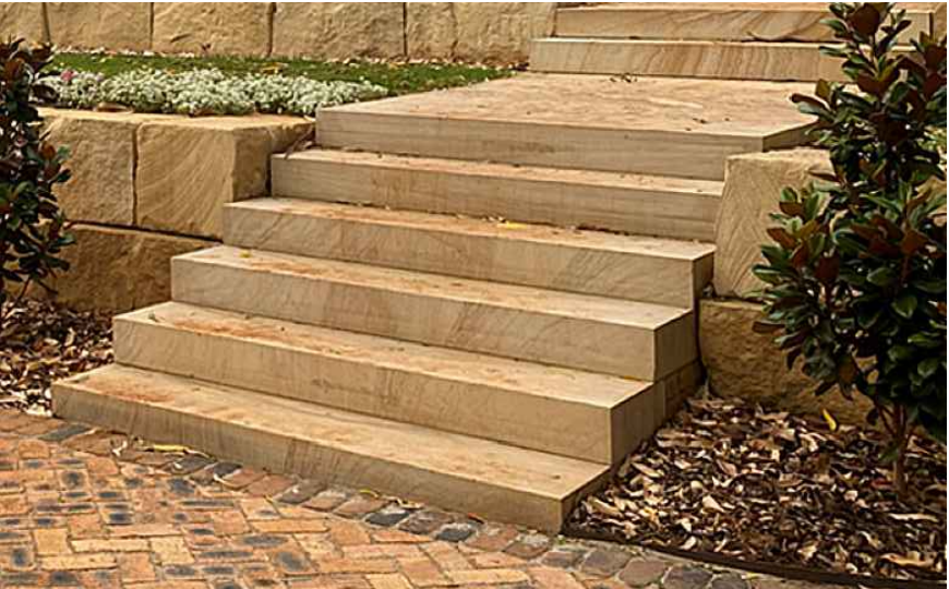
ST01 - SANDSTONE STAIRS ADJACENT TO SANDSTONE SEATING BLOCK
