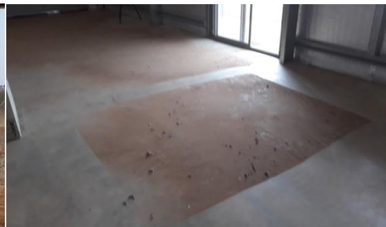
Clean up started (vacuum cleaner in use)
