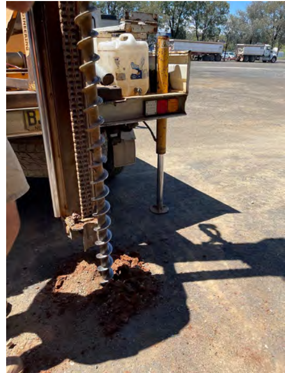
Figure 34. SP30 borehole displaying dry, natural soil beneath 700mm of road base/fill
