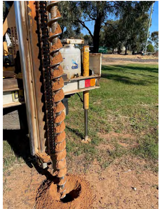
Figure 18. SP14 borehole displaying dry, natural soil
