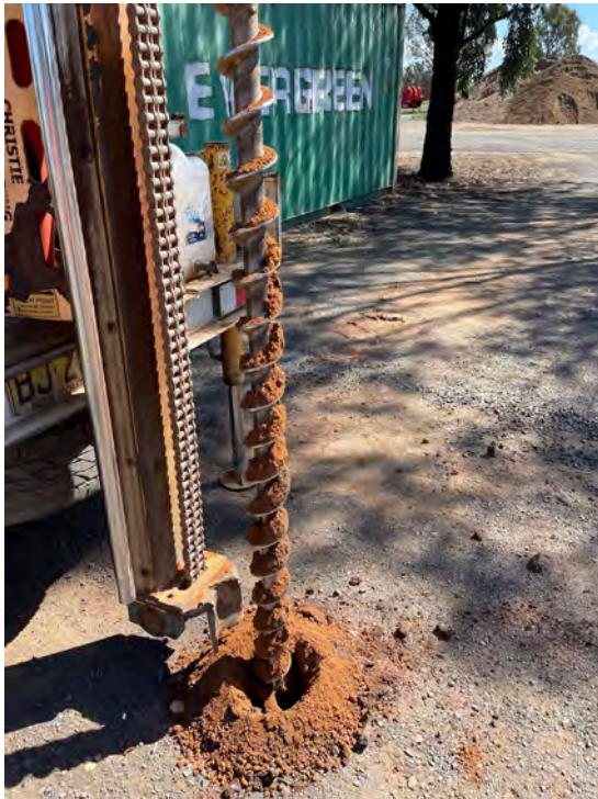
Figure 29. SP25 borehole displaying dry, natural soil
