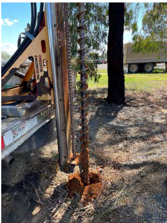
Figure 31. SP27 borehole displaying dry, natural soil
