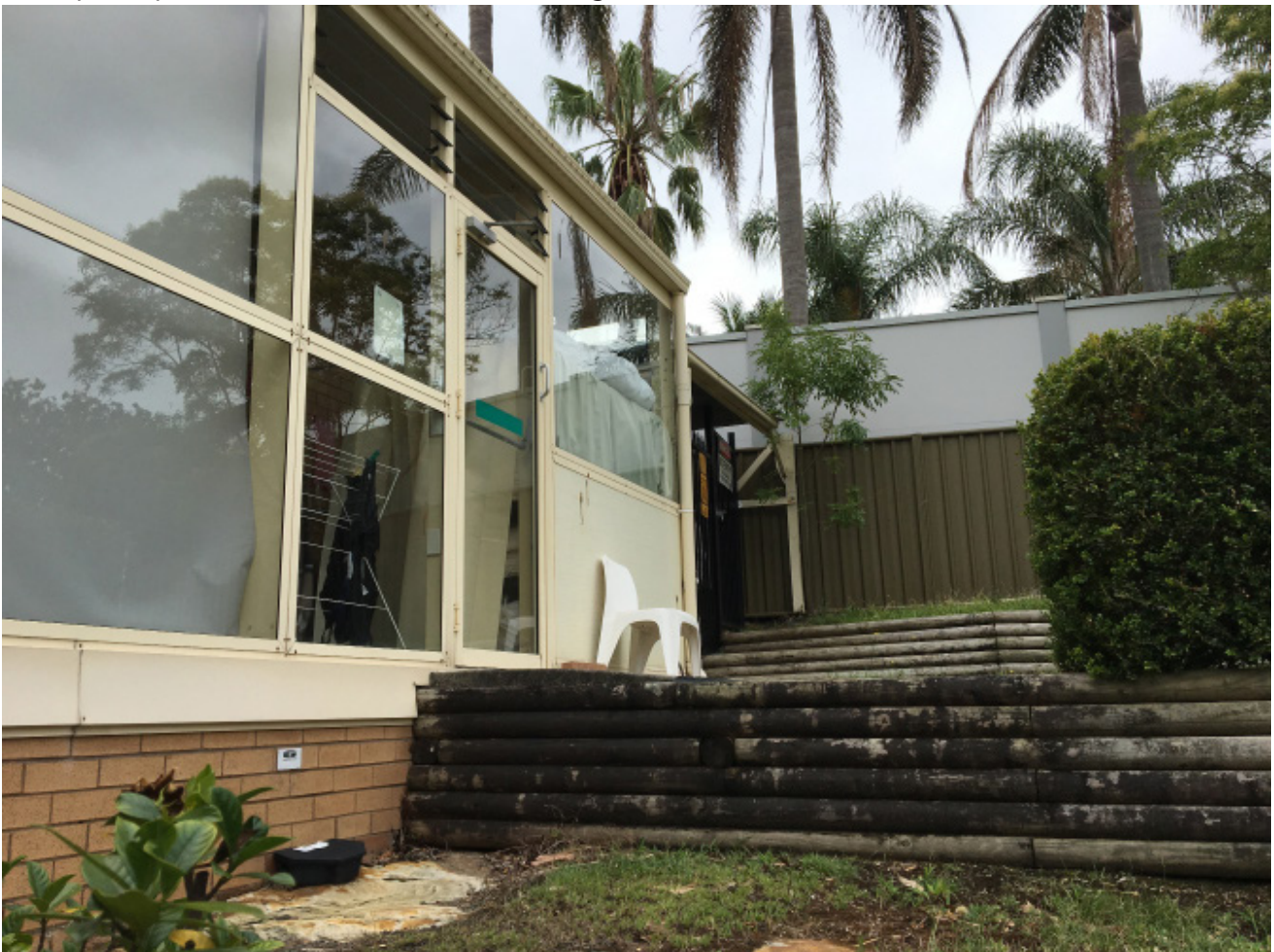
3.6 Open space at the rear of the building
