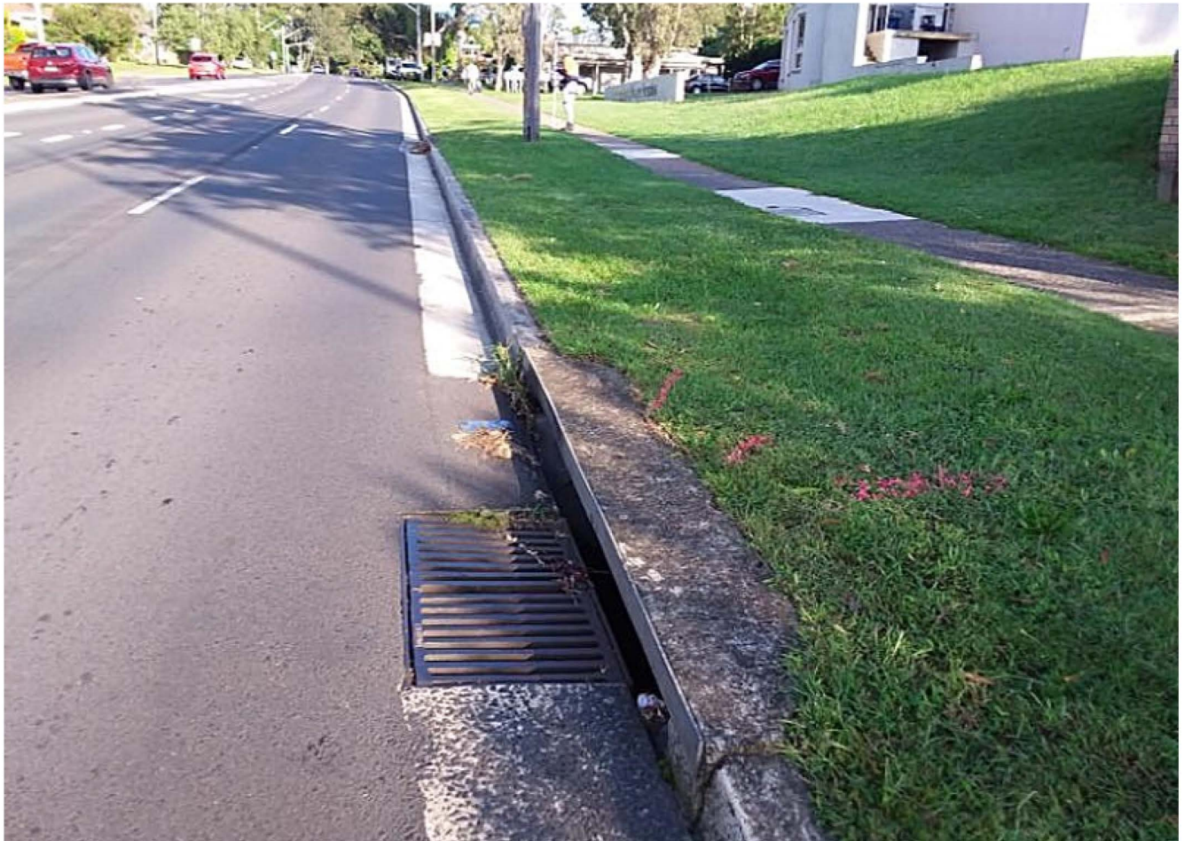
Pit in President Av, 2040mm invert from grate, appears to run straight to pit near cafe
