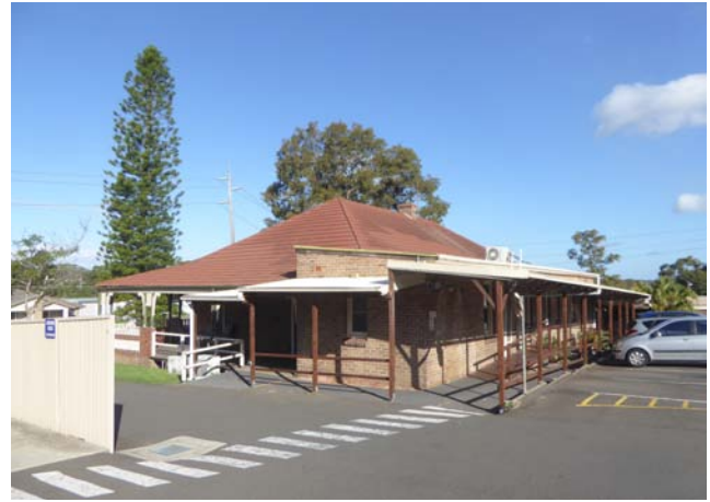
Figure 3.10 There is a skillion-roofed, single storey wing stretching across the back of the house, containing a number of services rooms. This wing has undergone extensive internal and external alterations. The covered walkway across the back of the building provides a form of accessible access for patients from the adjacent hospital accommodation.
