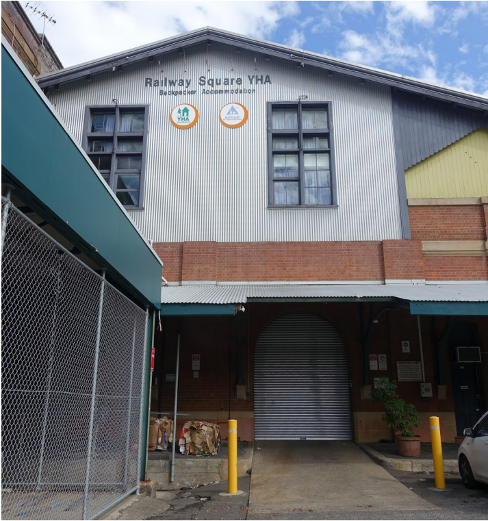
FIGURE 1 - PHOTO OF EXISTING FACADE
