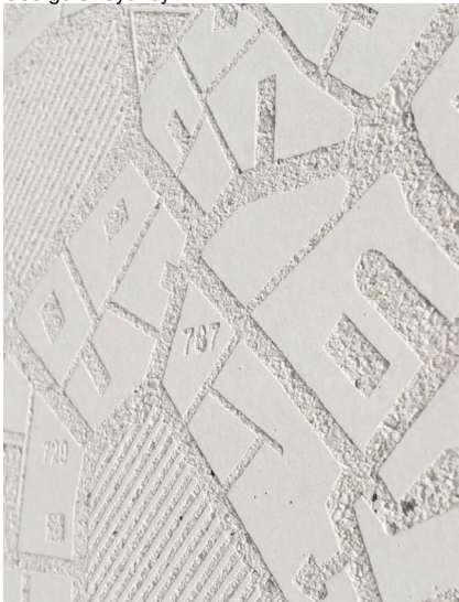
Graphic Concrete Woolside Health Centre Scotland
